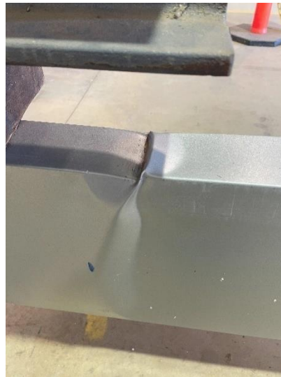
Figure 23 - Simply Supported Beam Failure Mode
