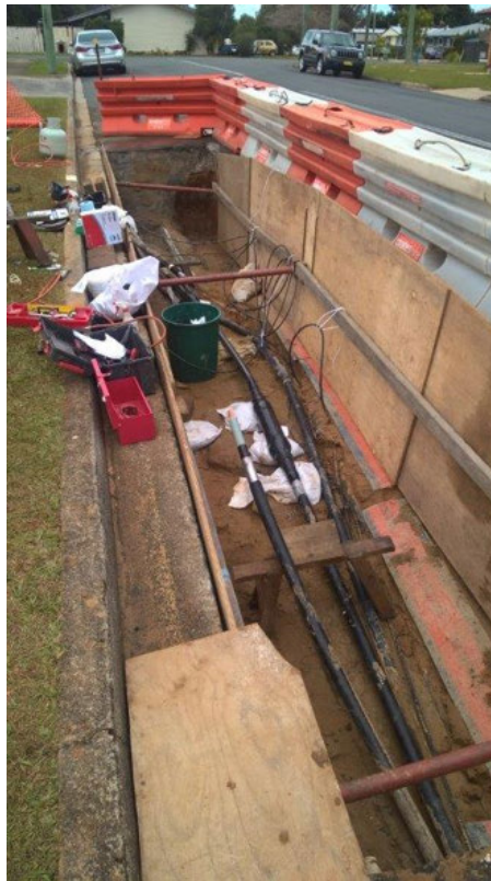
Figure 1.1: 33 kV cable joint bay (Source: Energex).
