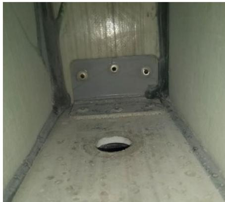
**Figure 3-2: SS angle bracket and rivets**
