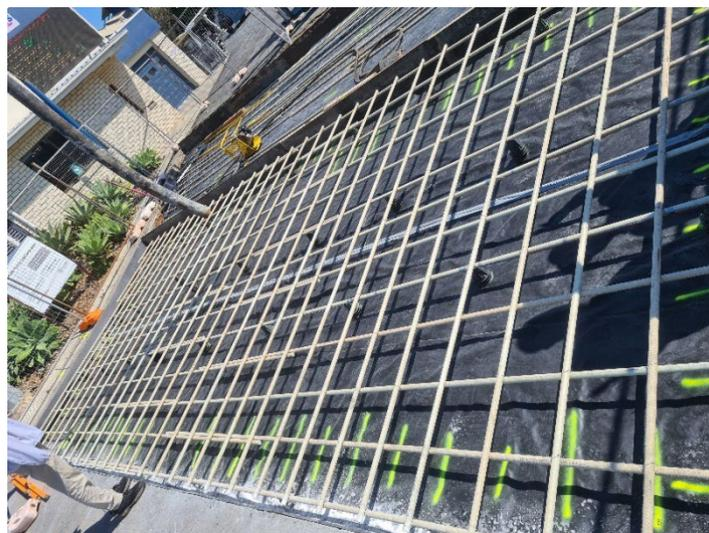
Figure 3.5: D24 mesh complete
