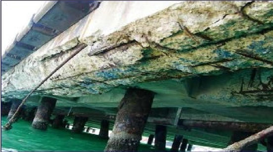
Figure 2.1: Reinforcement corrosion (Kodous 2021).
