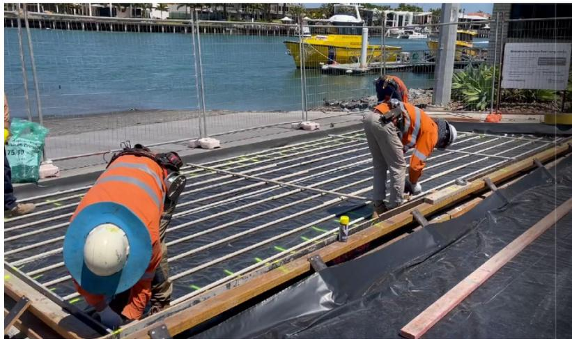
Figure 3.4: D24 mesh frame
