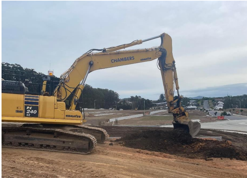
Figure 4.6: Excavator digging and moving material
