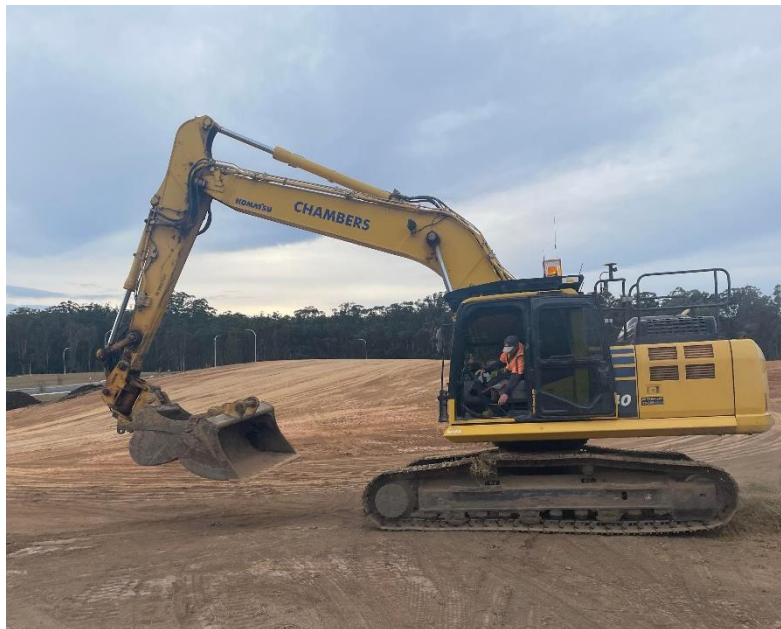
Figure 4.5: Excavator tracking 40m to pile of dirt
