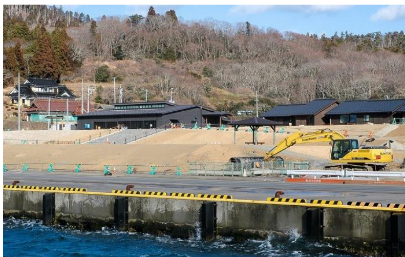
Figure 3.14: A 7.5m seawall in the fishing Port of Uranohama Oshima being covered in soil to maintain the natural look of the area (Satoru 2021)
