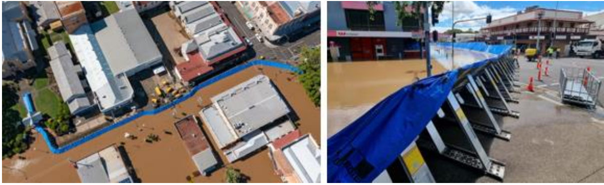
Figure 3.24: Temporary flood wall successfully holding back flood waters in Maryborough (Marie 2022)
