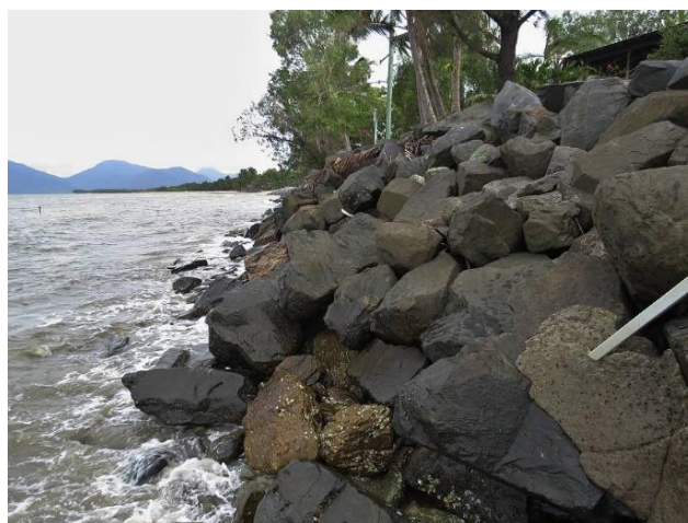
Figure 3.17: Old Machans Beach seawall. Badly eroded at the water's edge, with unsupported rocks that are close to collapse (Queensland Coast 2014)
