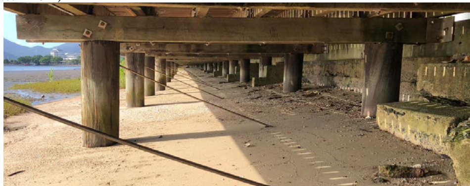
Figure 4.4(a): The new boardwalk was simply built over top of the old concrete wall, this wall is still what protects the southern part of Esplanade from erosion (O'Donoghue 2022)
