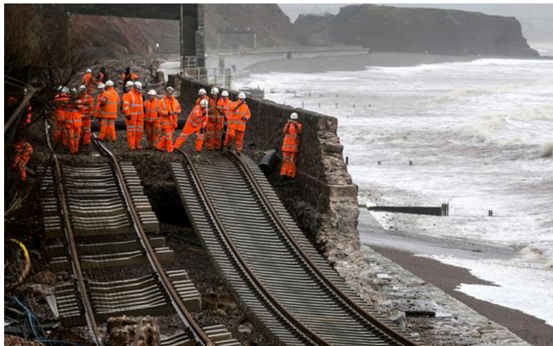
Figure 3.36: Storm waves caused the old Dawlish seawall to crumble (Channel 4 2014)
