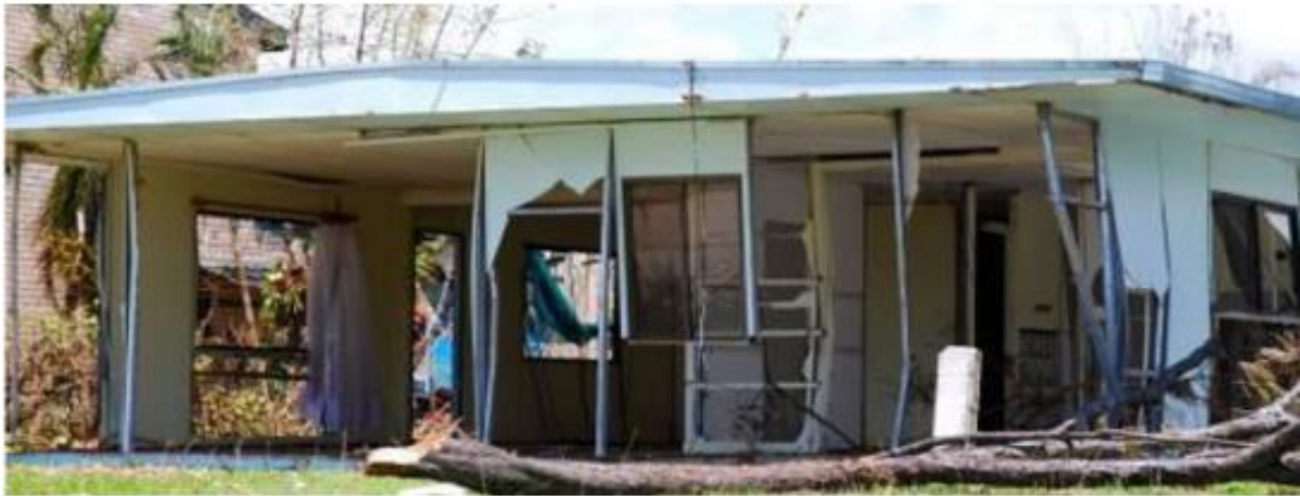
Figure 2.8(c): Damage to external walls on seaward side of house
