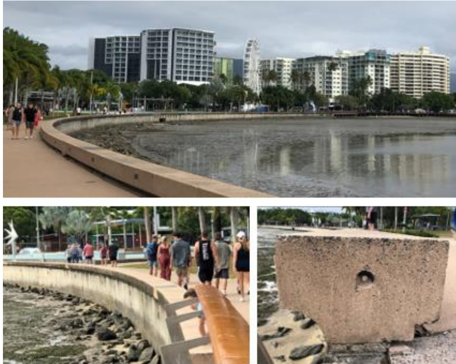
Figures 4.5: Vertical concrete seawall with a curved block on top protects a section of reclaimed land at the southern end of the Esplanade (O'Donoghue 2022)
