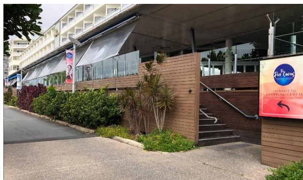
Figure 6: Ground floor of the Pier Shopping Centre raised 1.7m (O'Donoghue 2022)
