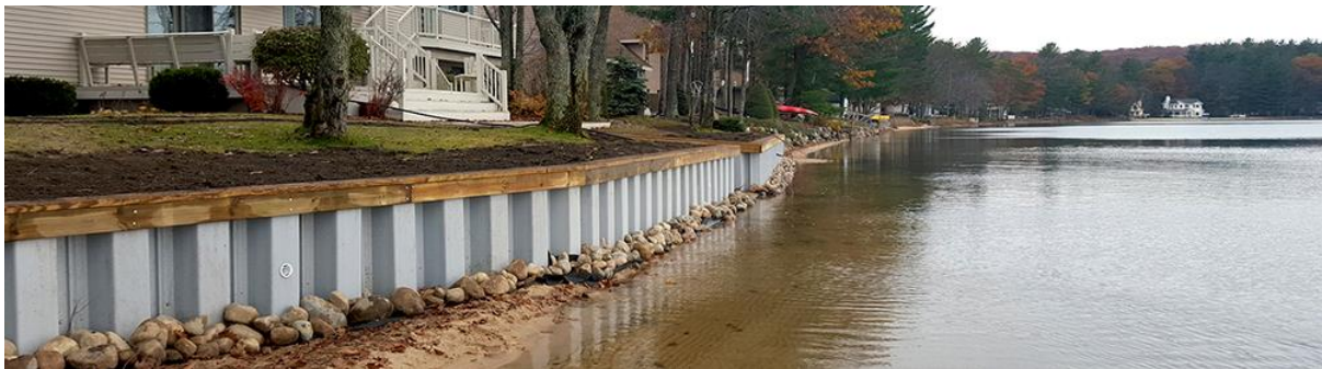
Figure 3.31: Small bulkheads protect against erosion in sheltered areas (Thaler Contracting 2022)
