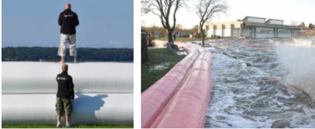
Figures 3.28(a) and 3.28(b): The system can be stacked to increase height and is suitable to protect from inundation from the sea (Bluemont 2022)
