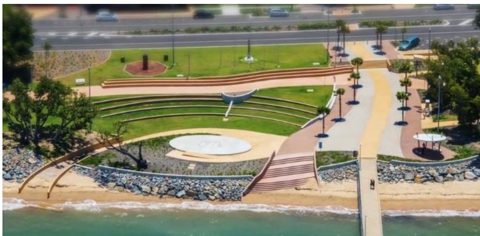
Figure 17: An attractive amphitheatre structure has been included as a feature that breaks up Cardwell's rip rap rock armour seawall (Watson 2014)
