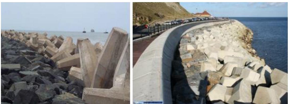
Figure 3.42(a): Combination wall of rip rap and tetrapods (Thaler Contracting 2022)
