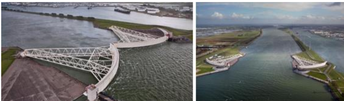
Figure 3.3: The 210 m Maeslantkering storm surge barrier allow ships to pass through the dam system into open ocean (Dutch Water Sector 2018 and Rijkswaterstaat 2022)
