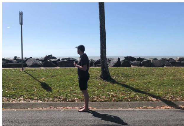
Figure 3: The Machans Beach seawall constructed in 2014, reclaimed about 6 m of land from the ocean and raised the ground level next to the wall in some areas by around 1 m (O’Donoghue 2022)
