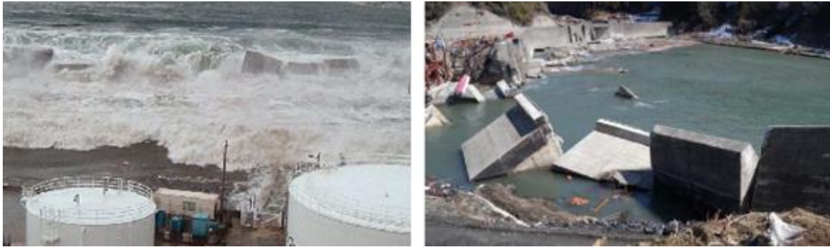
Figure 3.8(b) and 3.8(c): The seawall protecting the Fukushima Nuclear Power Plant disintegrated as soon as the tsunami hit and the failure of seawall at Ryoishi in Kamaishi (Daily Mail 2011 and PARI 2011)
