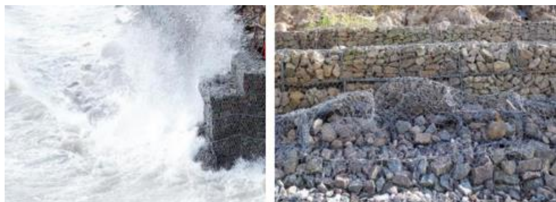
Figure 3.33(a) and 3.33(b): Wave action can destroy a gabion cage within a couple of years (Cherkasova 2019).
