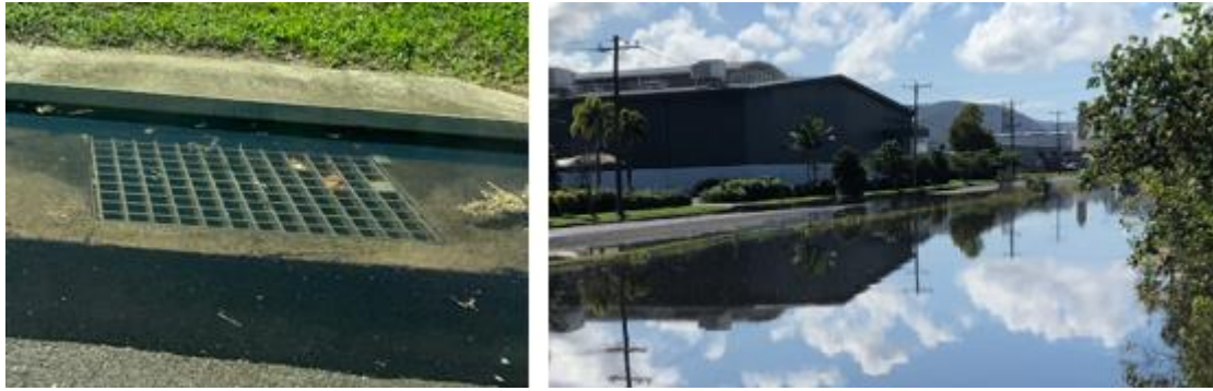
Figure 2.2(a) and 2.2(b): King tide tidal flows backing up through drainage systems, Cairns 2 January 2022 (Grant O'Donoghue 2022)
