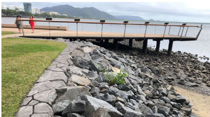
Figure 4.6: Rip rap revetment with a decorative concrete edge fronts some sections of the reclaimed land at the southern end of the Esplanade (O'Donoghue 2022)
