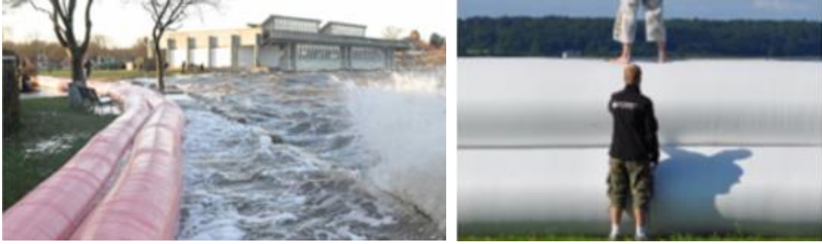
Figures 14(a) and 14(b): The NoFloods mobile flood barrier can be quickly constructed to protect from large king tides or cyclonic storm surge (Bluemont 2022)
