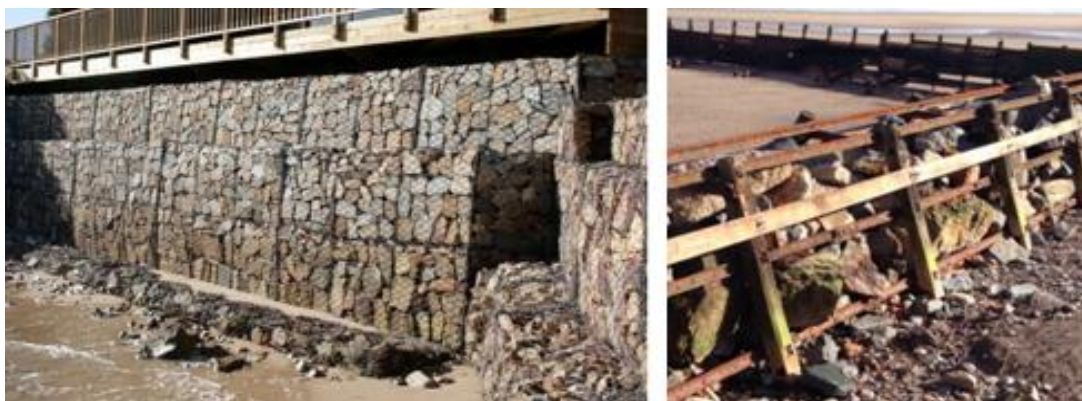
Figure 3.32(a) and 3.32(b): Gabion walls made out of stacked wire cages and recycled railway lines (Aathaworld 2022 and Coasts 2022)
