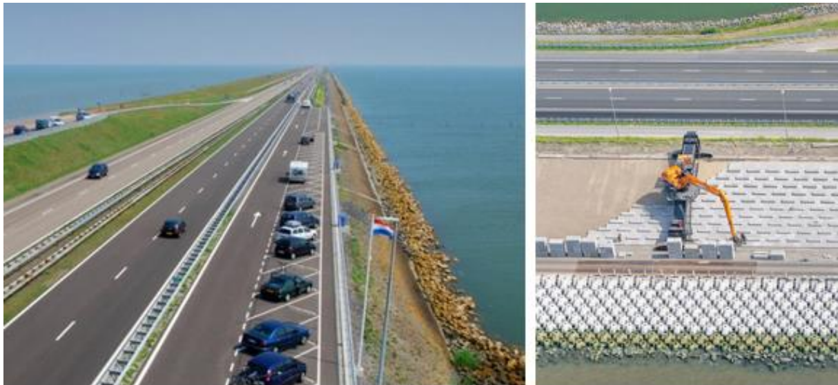
Figure 3.5: The 32 km long Afsluitdijk dyke is being raised by 2 m and reinforced with a layer of concrete armour (Tegg 2018 and Reina 2021)
