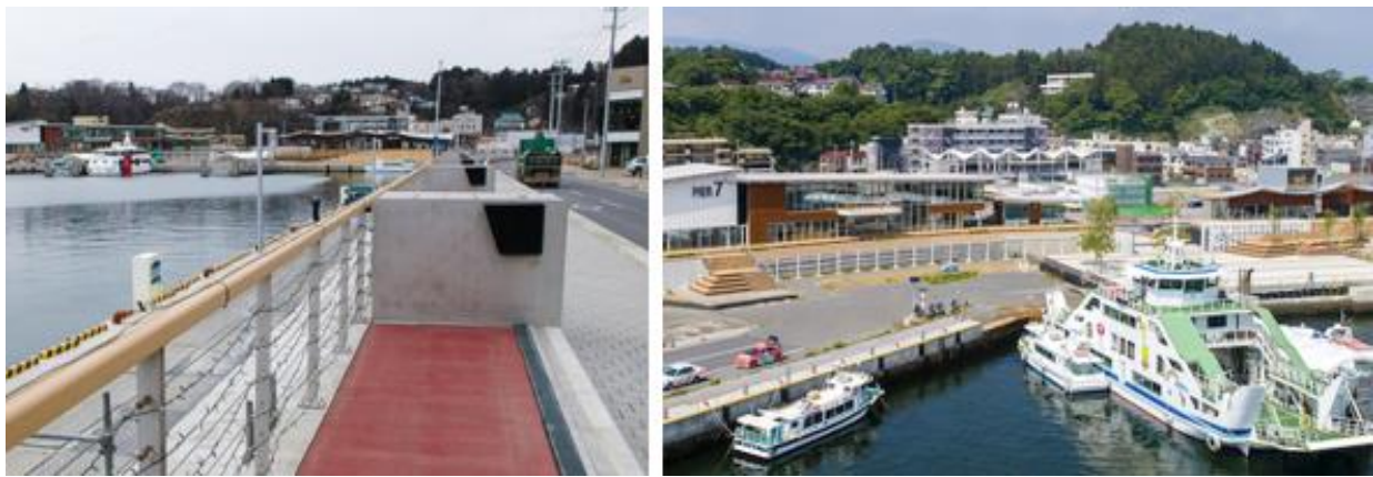
Figure 3.15(a): Naiwan seawall has an additional 1m flap (red) which is automatically raised by water pressure in the event of a tsunami (Satoru 2021)
