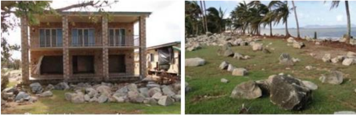
Figures 2.8(a) and 2.8(b): Damage to the bottom level of a house at Tully Heads where armour rocks from the seawall have been washed onto the lawn by the wave energy of Tropical Cyclone Yasi's 5.33 metre storm surge.
