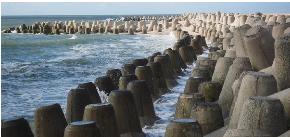
Figure 3.40: Tetrapod mound wall (Southern Dredging & Marine 2022)
