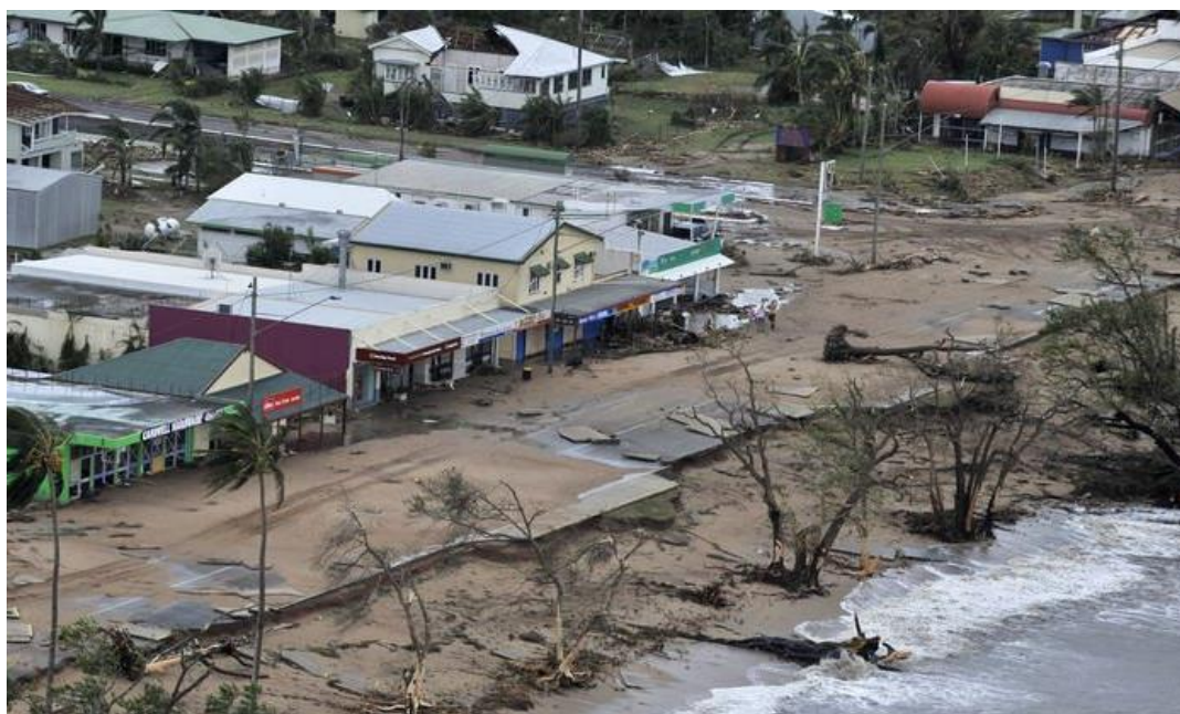
Figure 2.6: Damage to Cardwell foreshore with part of the Bruce Highway washed into the ocean by the storm surge that accompanied Cyclone Yasi in 2011 (Dept. Science. Qld Govt Cyclone Yasi Report, 2012)
