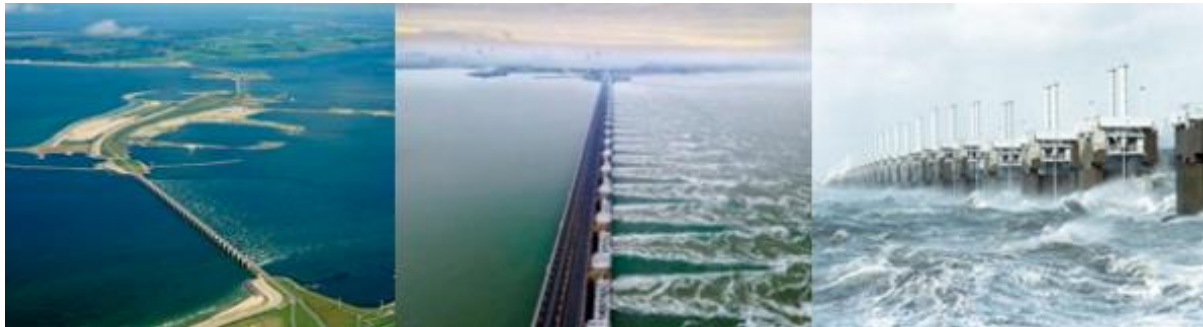
Figure 3.2: The 9 km Oosterschelderkering barrier includes 4 km's of sluice gates that allow natural water flow but can be closed during extreme storm events (Deltawerken 2022)
