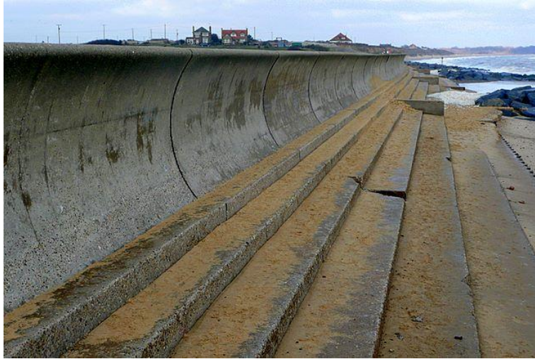
Figure 3.35: Curved seawall with stepped base at Southwold UK (Horn 2008)
