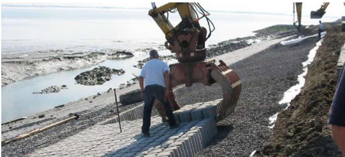
Figure 3.41: Construction of concrete block armour on a Netherlands revetment (Breteler et al. 2014)
