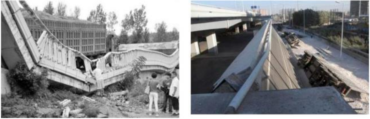
Figure 5: Bridge failures due to overload (Zhang et al, 2022)
