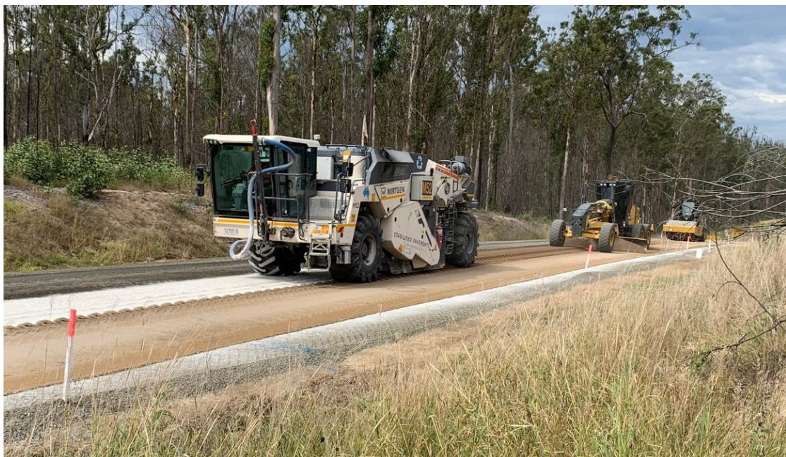
Figure 4. 4 - Stabilisation of the Braemar project (Source: Shaun Perkins 2020)
