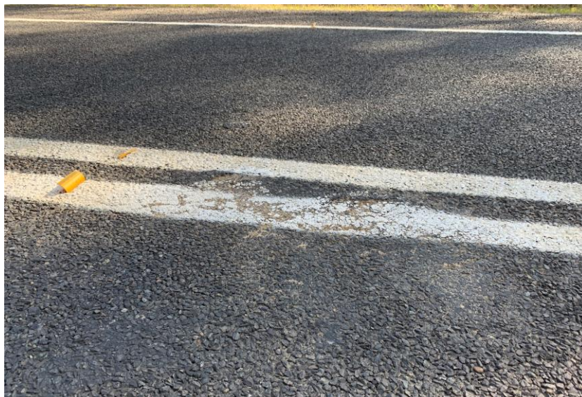
Figure 5. 3 - Shoving on the centerline of the Braemar project (Source: Shaun Perkins 2022)
