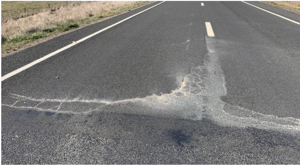
Figure 5. 6 – Cracking at western pavement interface of the Boree project (Source: Shaun Perkins 2022)
