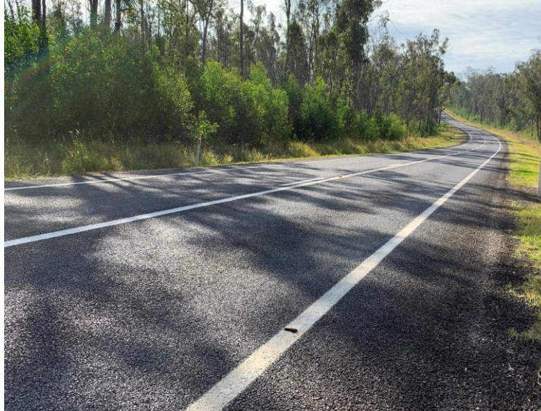
Figure 5. 4 - S45R final seal of Braemar project as preventative maintenance (Source: Shaun Perkins 2022)
