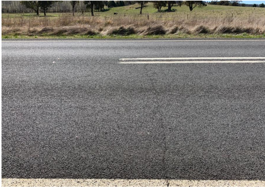
Figure 5. 5 – Transverse shrinkage cracking at the Boree project (Source: Shaun Perkins 2022)
