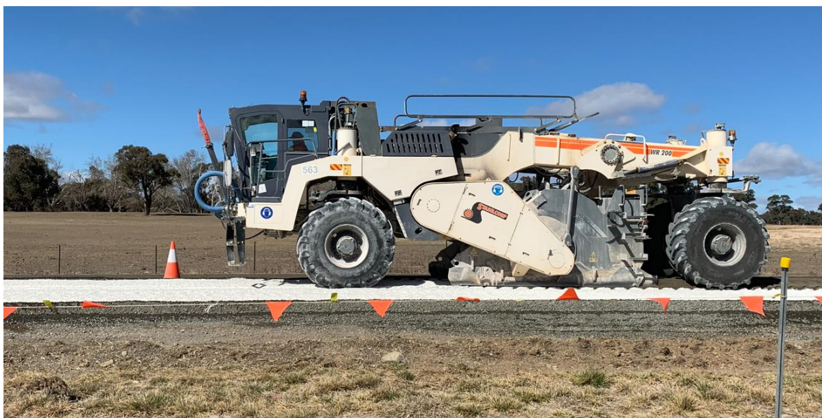
Figure 4. 3 – Stabilisation of the Boree project (Source: Shaun Perkins 2020)
