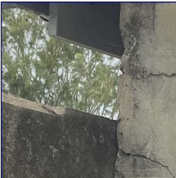
Figure 3: Spall and crack image with background noise Image courtesy of: A. Bourke
