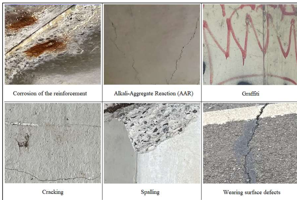
Figure 1: Various defect types identified during field inspections Images courtesy of: A. Bourke
