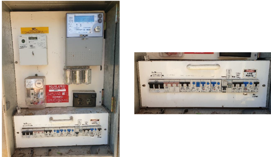
Figure 10: Site 3 photos: MSB (left) and sub-circuits (right)
