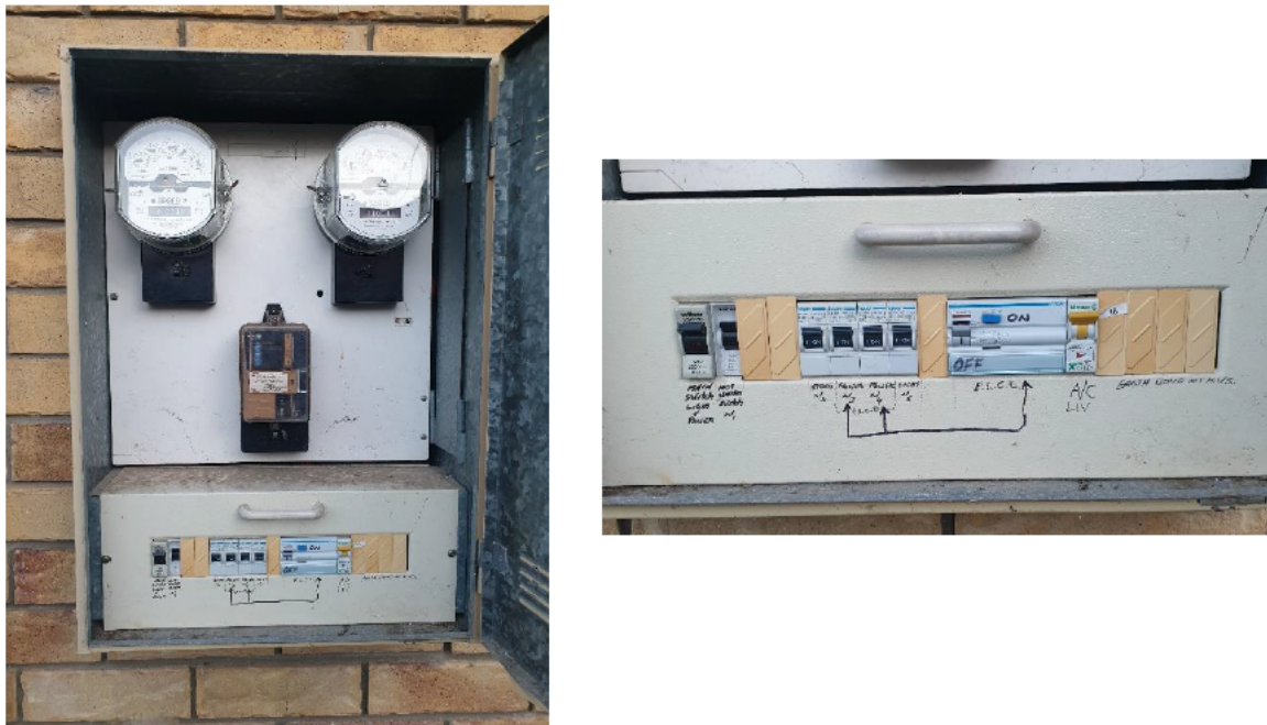
Figure 8: Site 1 photos: MSB (left) and sub-circuits (right)
