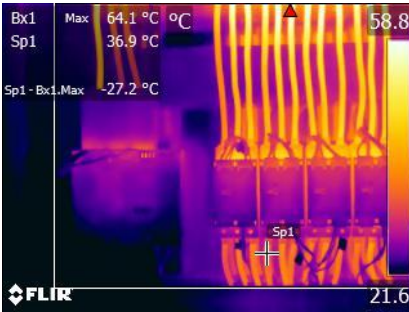
Figure 5.19 Water-based Amusement Ride 1 thermal image of conductors
