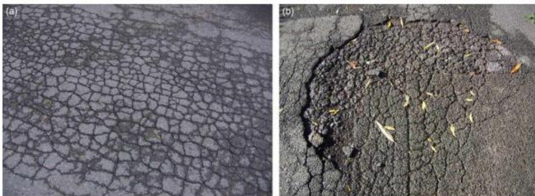
Figure 4 Examples of crocodile cracking (Croll 2009).
