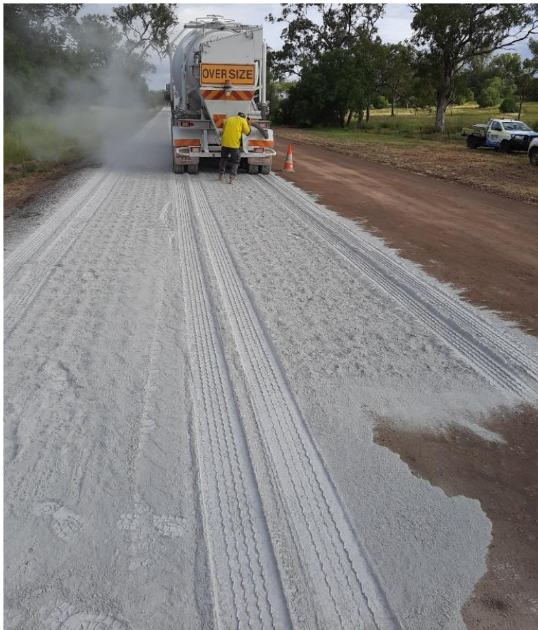
Figure 1 Cement powder spreading.
