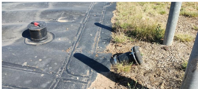
Figure 13: Sludge draw off and inspection port.
