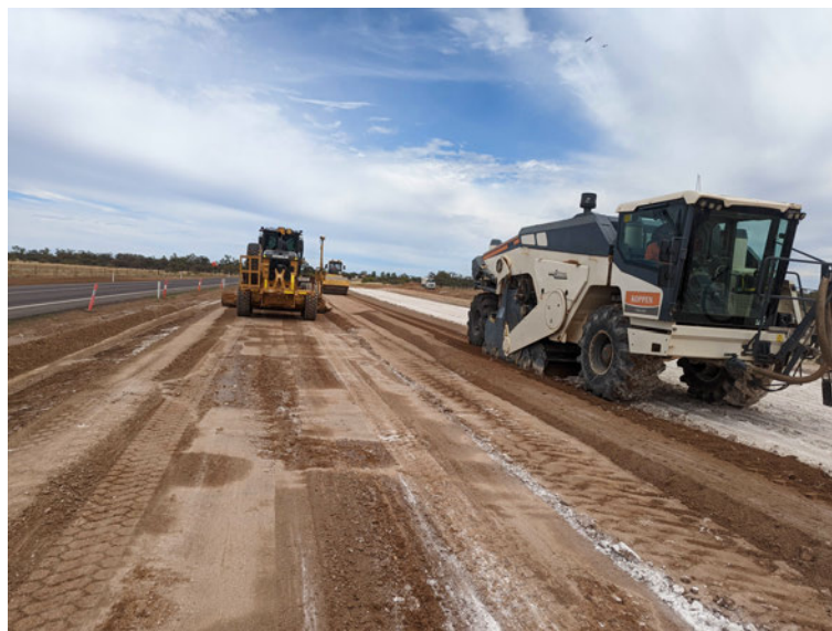
Figure 2.7: Slaked lime being incorporated into the subgrade using a Wirtgen soil stabiliser. (R Kashanov 2022, personal photograph, 1 October)
