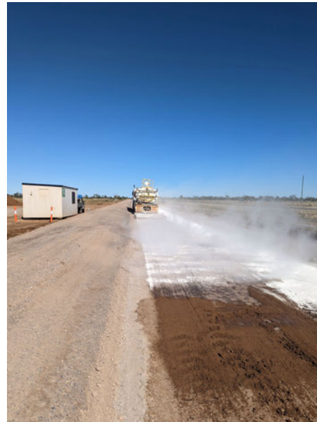
Figure 2.6: Quicklime being slaked with a modified water tanker. (R Kashanov 2022, personal photograph, 9 July)
