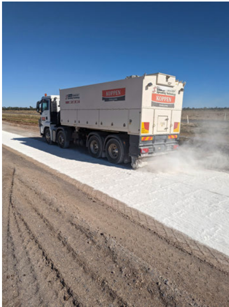
Figure 2.5: Quicklime being spread with a spreader truck. (R Kashanov 2022, personal photograph, 9 July)
