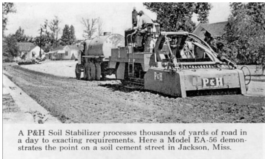
Figure 2.3: Excerpt from an unknown news publication showing a P&H stabilisation machine, reproduced from the collection of historic photos and documents produced by or related to the Harnischfeger, P&H or JoyGlobal prepared by Ray (2017).
