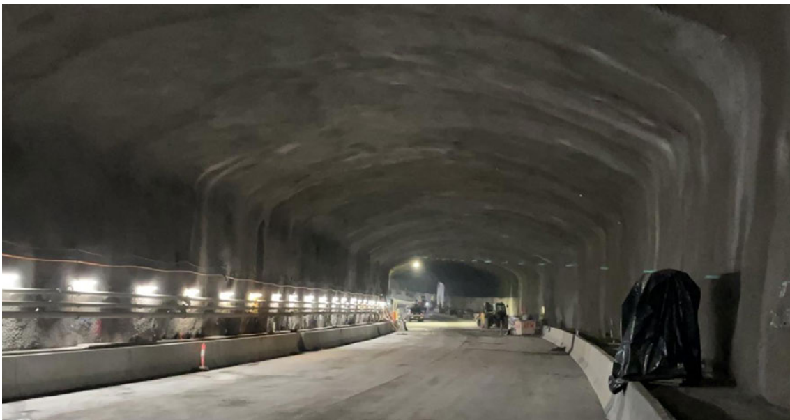
Figure 2 Tunnel profile - horse shoe shape cut in sandstone substrate.
