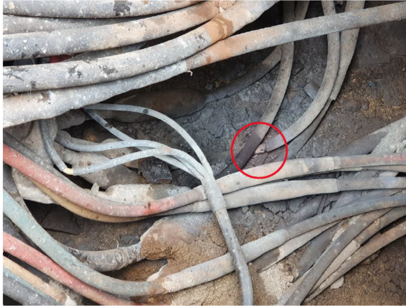
Figure 23 Photograph of Fault Within Pit for Site 1
