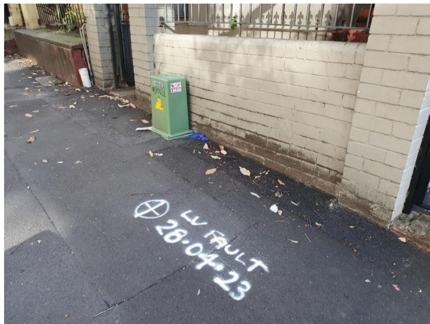
Figure 27 Photograph of Fault Located Adjacent to Low Voltage Pillar
