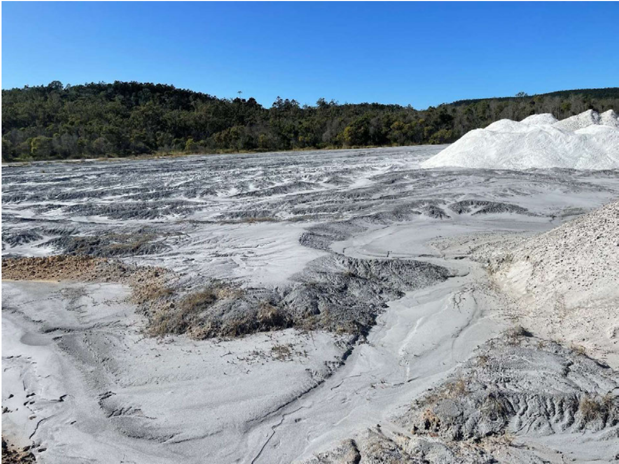
Figure 1.2 Image taken while sampling HA at Tarong Power Station showing the surface of the CCP Dam and on right hand side stockpiled BA.
