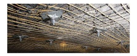
Figure 2.4: Roof support in an underground coal mine used for strata support, also can be used for lifting pieces of equipment (Mining Weekly 2023).
