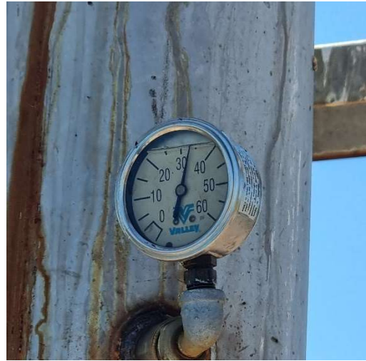
Figure 6.2: Pressure Gauge on Standpipe, Source Student
