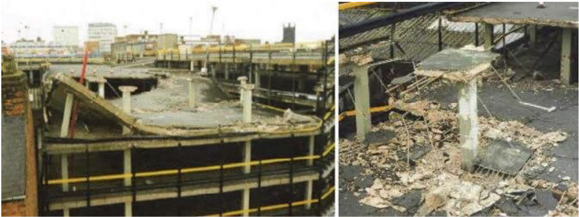
Figure 2: Floor collapse of Wolverhampton Parking due to punching shear failure (Wood, 2003)
