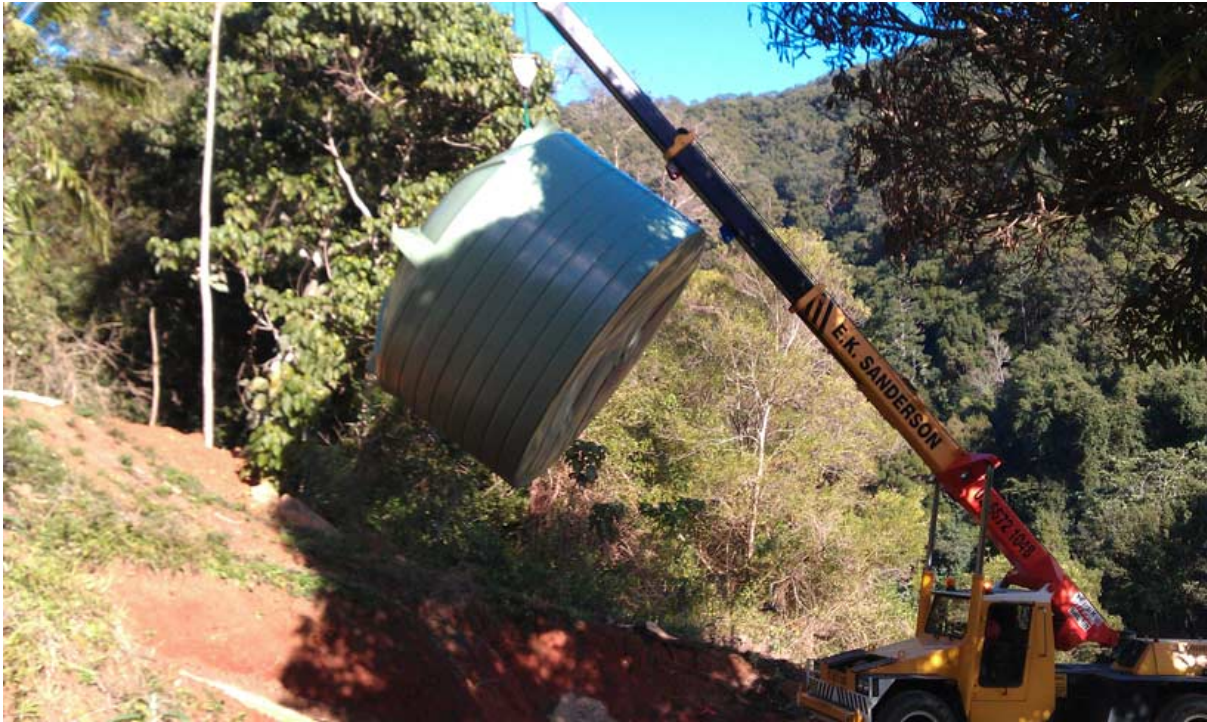
Figure 39 – Crane lifting rainwater tank
