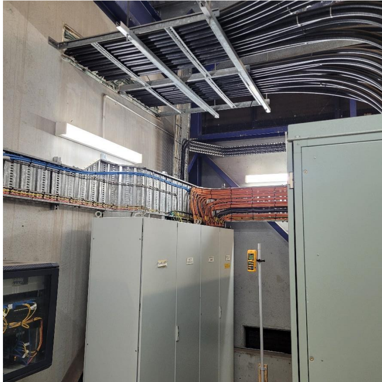
Figure 4.4.1.2 SCADA RTU installed directly beneath cables.
