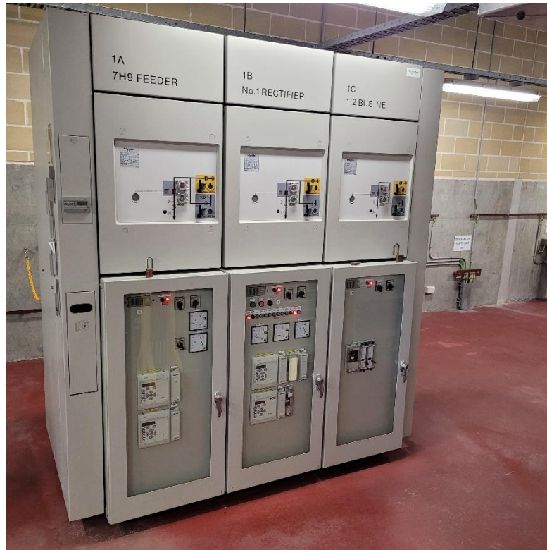
Figure 2.2 Typical Sydney Trains 33kV GIS Bus Section
