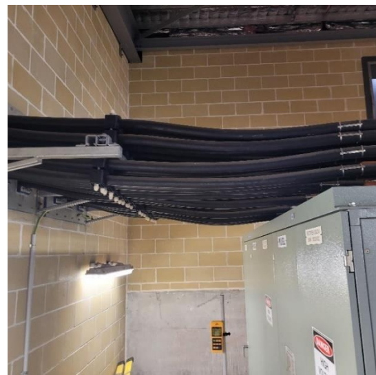
Figure 4.3.1b EMF meter positioned under 600V AC cables.
