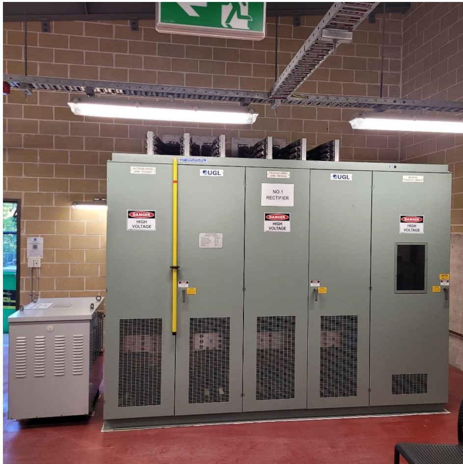
Figure 4.3.8.1 Front of Rectifier Diode Unit.
