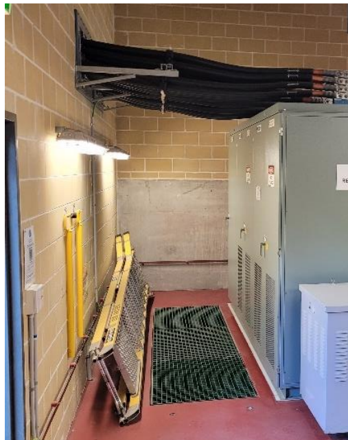
Figure 4.6.3 Storage of operating handles and ladders under 600V AC cables
