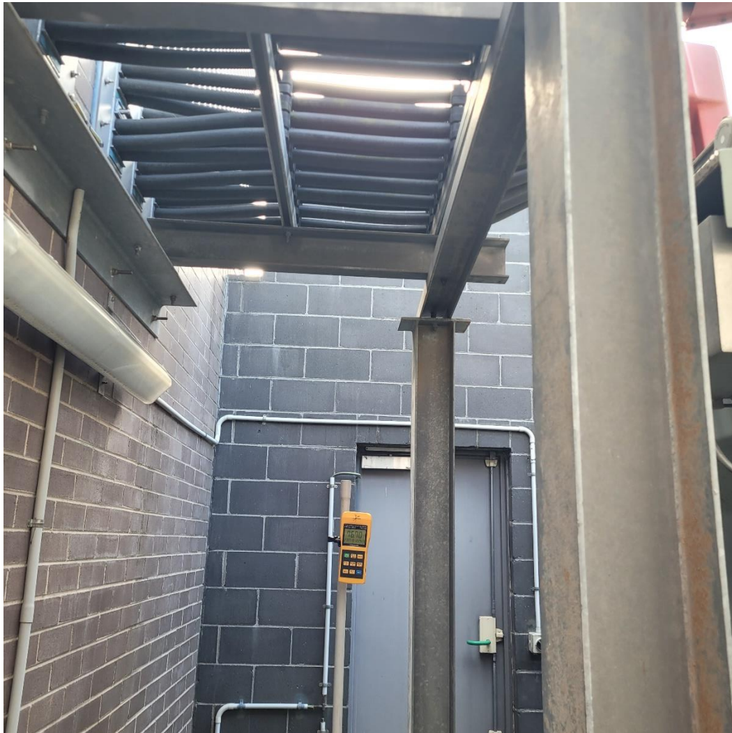
Figure 4.5.2.1 Yagoona Under 600V AC Cables in Transformer Yard.
