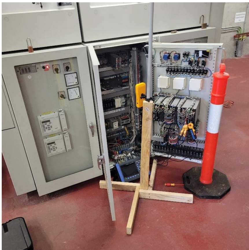
Figure 4.3.3 Meter located in front of ACCB.
