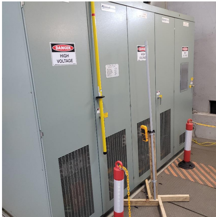
Figure 4.4.4.1 Magnetic Field Meter Front Side of Diode Unit.
