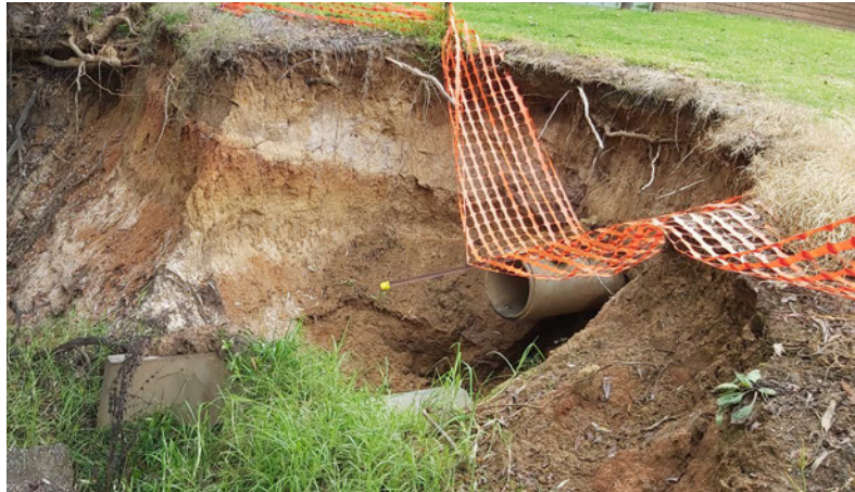
Figure 2.6: Severe scouring at a culvert outlet.
