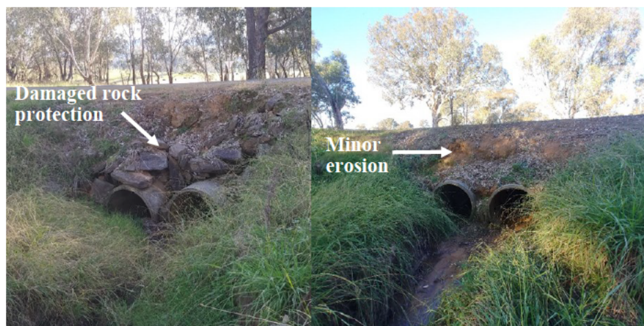
Figure 4.5: Damage to a culvert on the upstream (left) and downstream (right) side.
