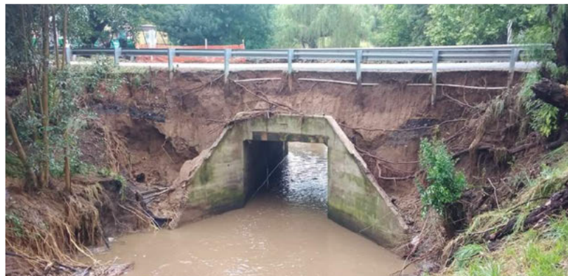
Figure 2.5: Embankment erosion on the downstream side of a culvert.
