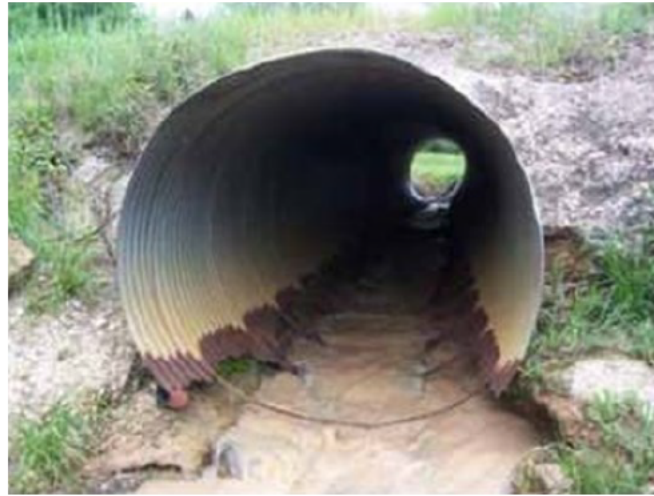
Figure 2.2 A CMP culvert with corrosion damage (Haghani & Yang 2016).
