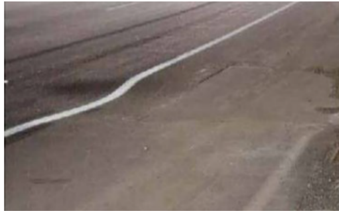
Figure 2.4: Road settlement due to piping (Piratla, Jin & Yazdekhashti 2019).
