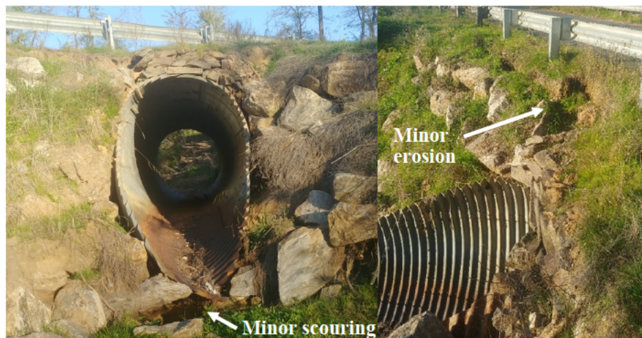
Figure 4.7: Minor damage to a CMP culvert on the downstream side.
