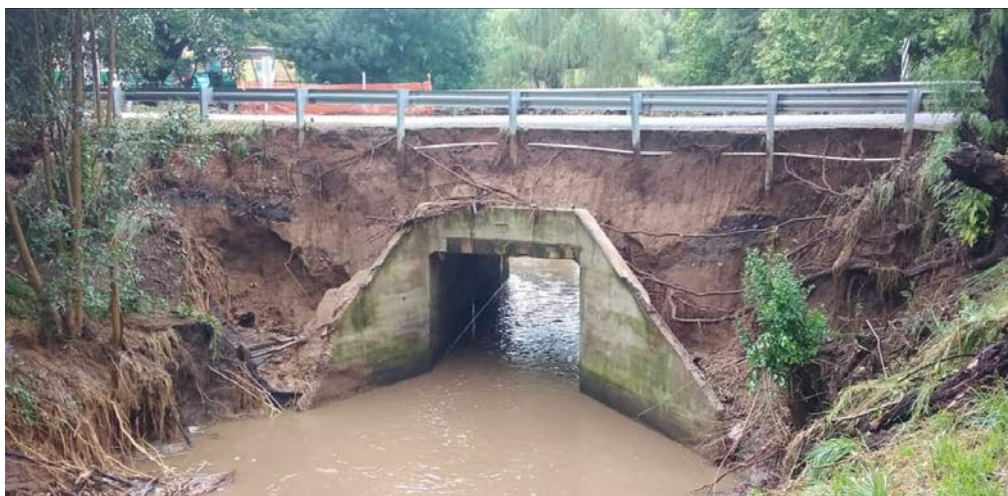
Figure 6.4: A heavily damaged box culvert analysed during the field investigation.
