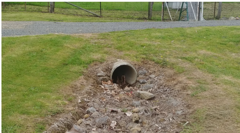
Figure 1.1: A small driveway culvert.
