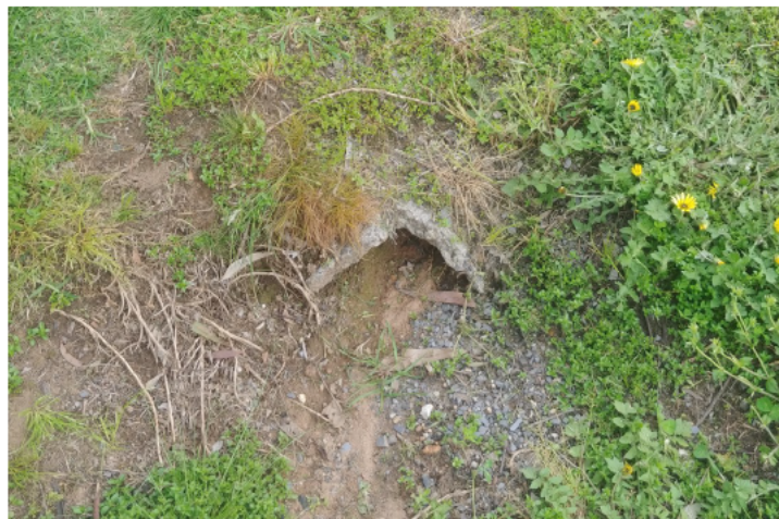
Figure 2.3: Mechanical damage on an exposed driveway culvert.
