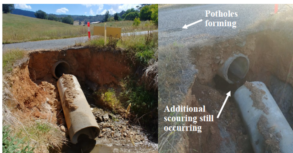
Figure 4.6: Scouring damage to a culvert on the downstream side.
