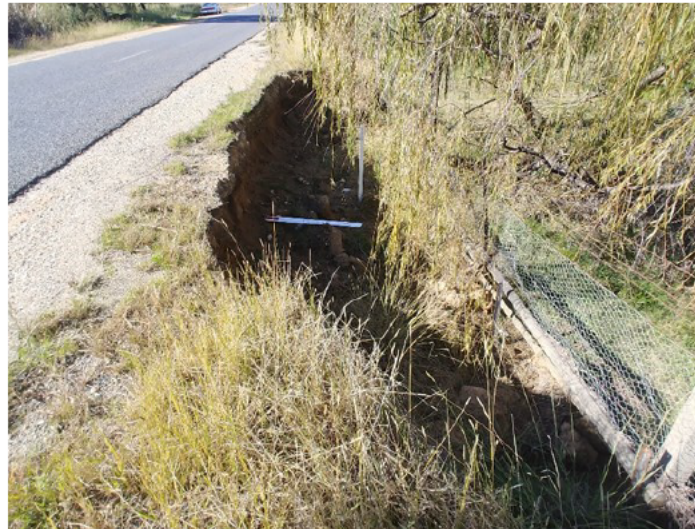
Figure 4.9: Erosion damage adjacent to culvert 4 outlet.
