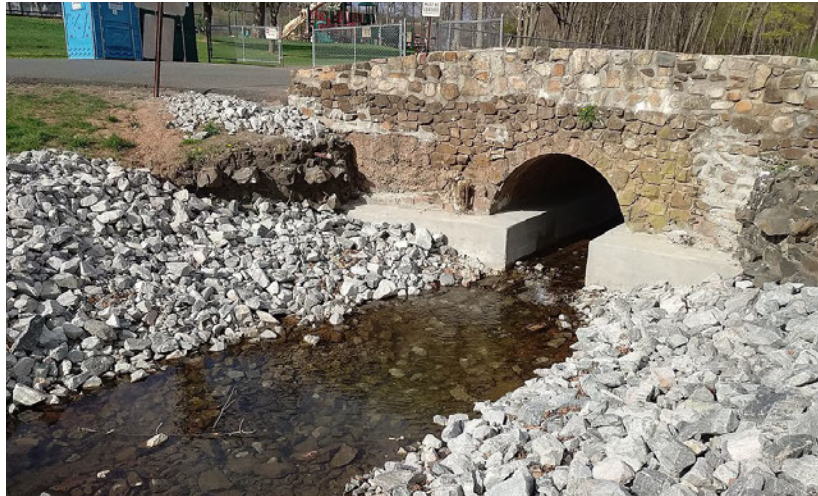
Figure 2.8: Riprap Protection at a culvert outlet (Wikipedia 2022).
