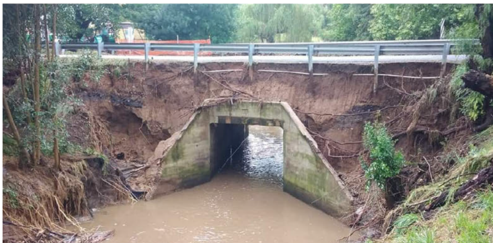
Figure 4.3: A major culvert failure in Bethanga, Victoria.
