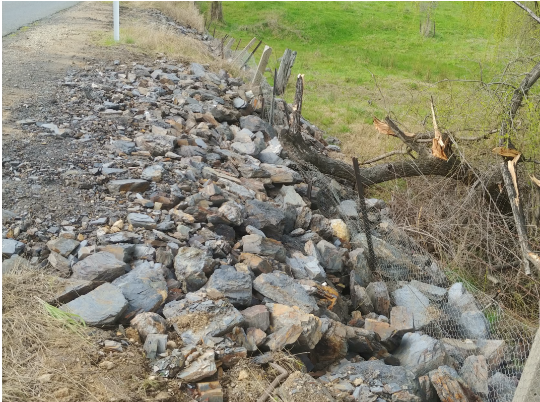
Figure 6.12: Culvert repair using crushed rock and rip rap.
