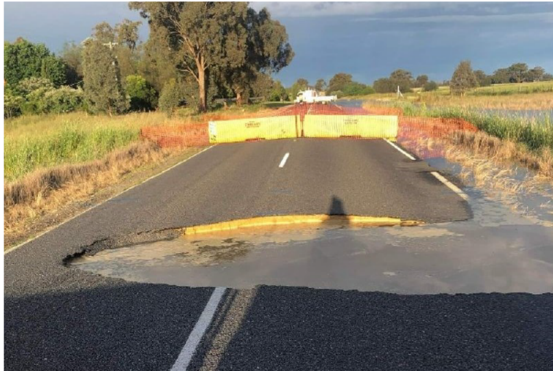
Figure 4.2: Culvert failure near Rutherglen, Victoria (Indigo Shire Council 2022).
