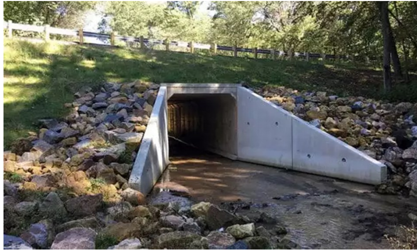
Figure 1.2: A larger box culvert supporting a roadway (Dream Civil 2022).
