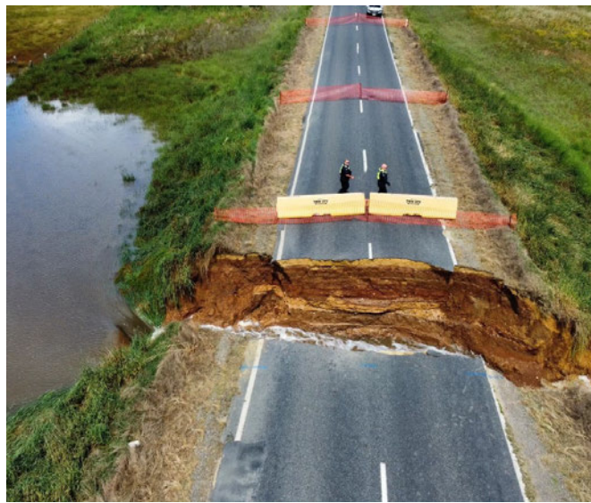
Figure 4.1: Culvert failure near Rutherglen, Victoria (Indigo Shire Council 2022).
