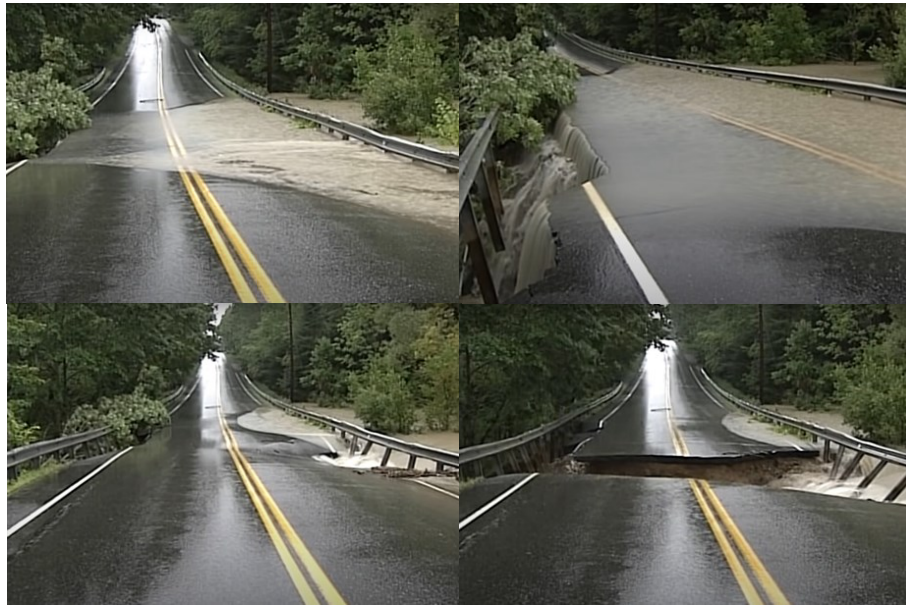
Figure 2.7: Progressive failure of an overtopping culvert (Vermont Local Roads 2012).
