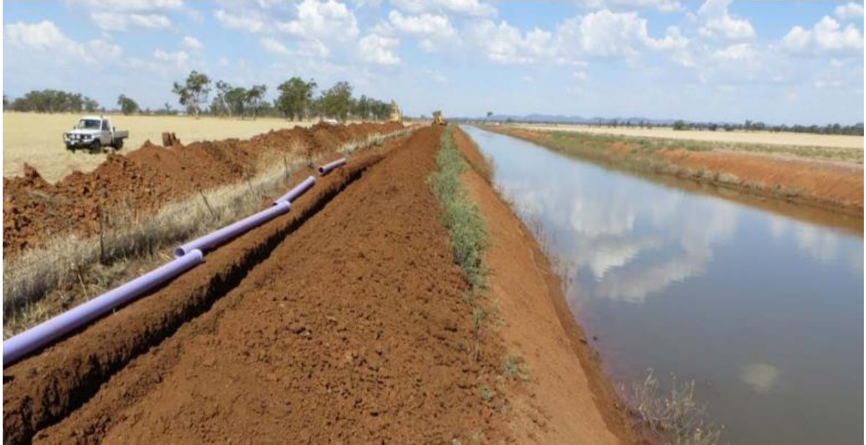
Figure 3-4 Construction of Stock and Domestic Pipeline by Mitchell Water (McBurnie 2017)
