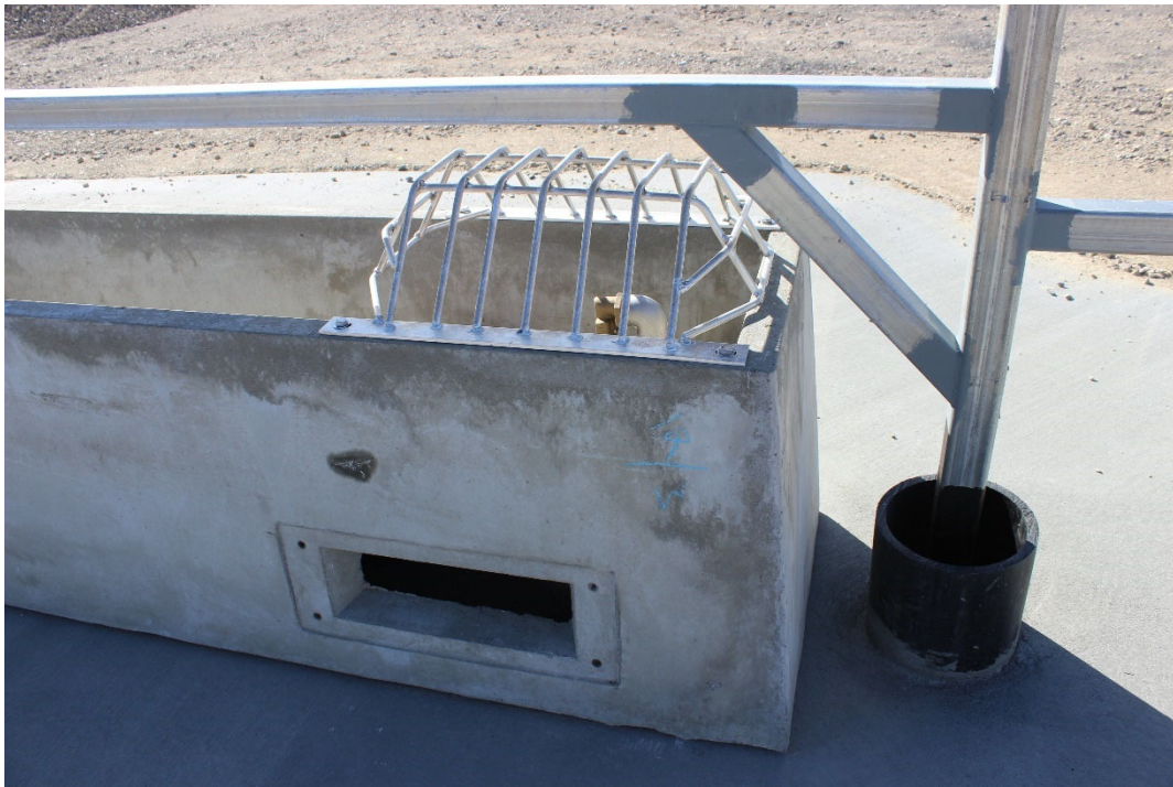
Figure 69: Conventional Concrete Trough – Typical wire cage float protection (RDC Engineers Pty Ltd)
