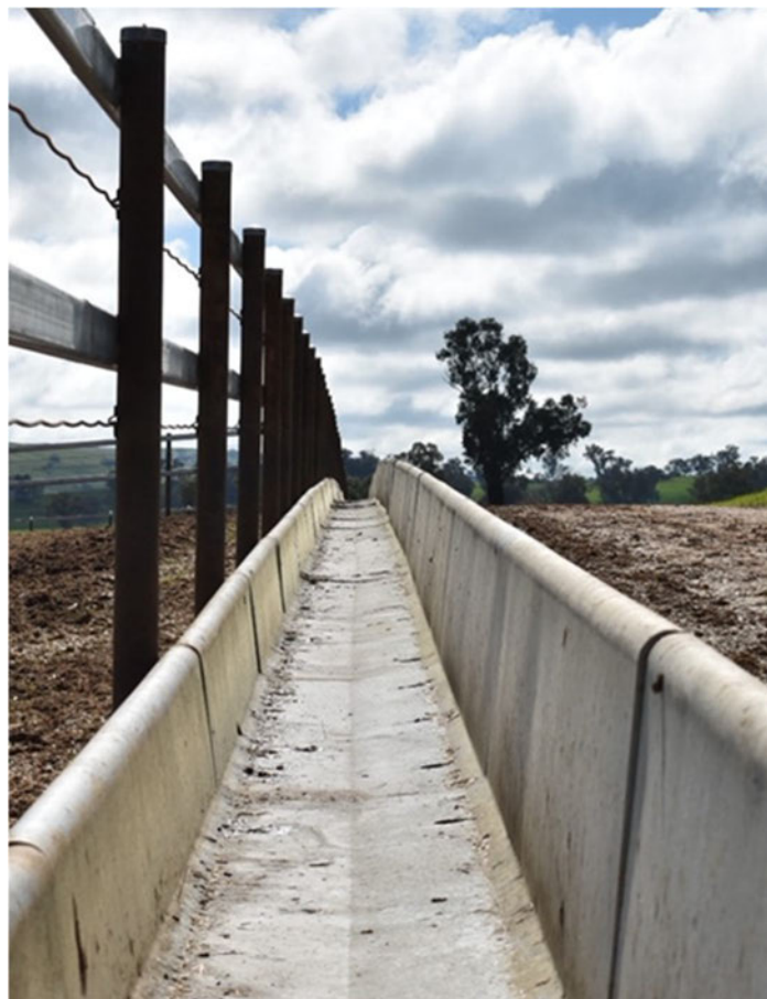
Figure 11: Australian Intensive Feeding – Typical open feed bunk (Conron Stock Crete, 2024)
