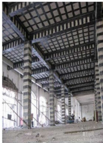
Figure 1.2. Bidirectional/Unidirectional/Mixed knitted/Construction reinforcement carbon fibre fabrics
