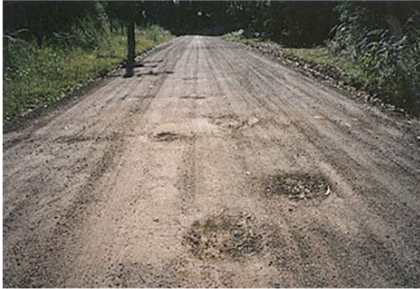
Figure 10 – Potholing Defects (Austroads, 2009, pp. 54)
