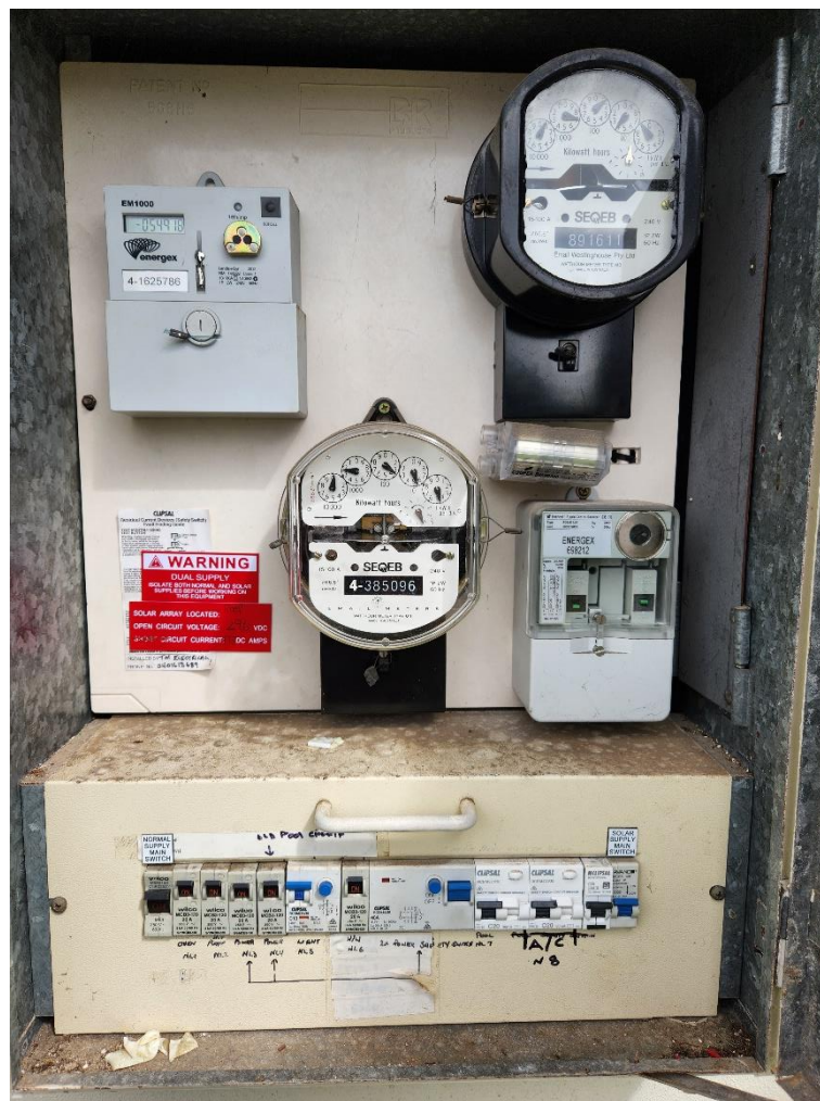
Figure 11. A residential switchboard showing individual protective devices and metering equipment.
