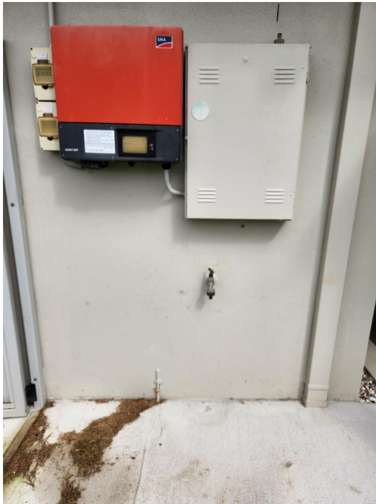
Figure 16. A 5kW grid connected inverter adjacent a residential switchboard.
