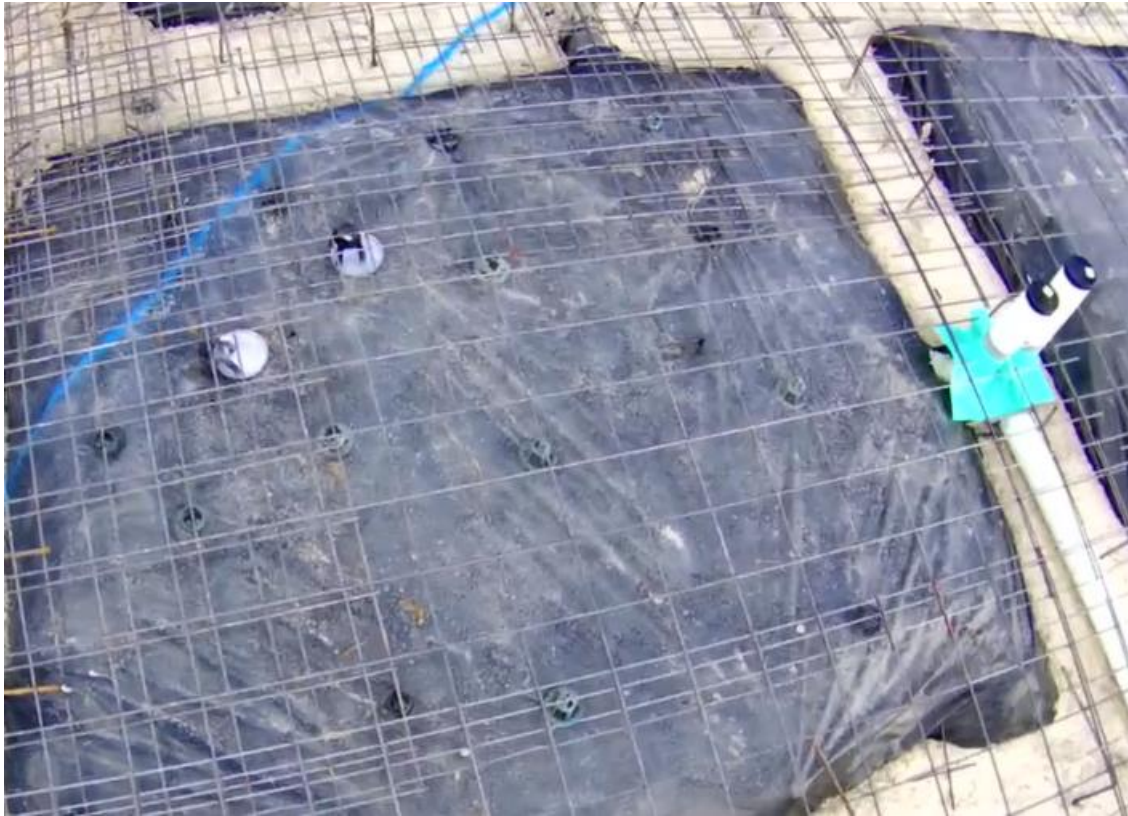
Figure 25 - Suitable Membrane Condition and Pipework Protection
