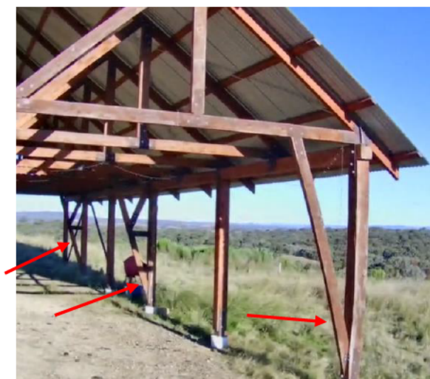
Figure 27 - Brace Sets and Columns
