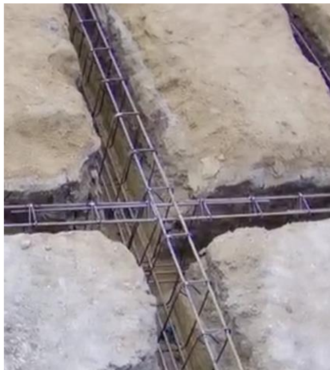
Figure 18 - Detailed Image of Foundation Intersection
