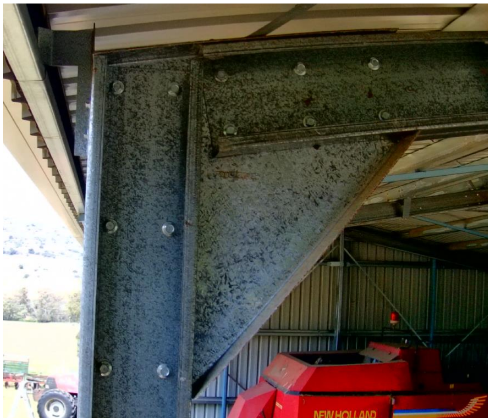
Figure 35 - Rafter to Column Connection
