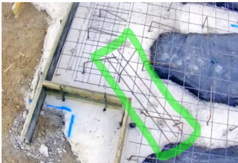
Figure 22 - Re-entrant Corner Slab Bars
