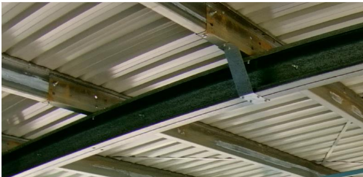
Figure 33 - Purlin Lap and Bolt Arrangement
