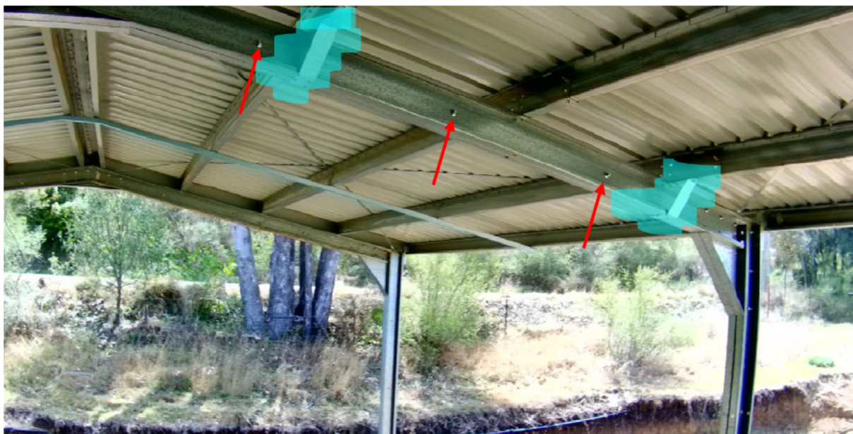
Figure 31 - Flybraces and Portal Rafters
