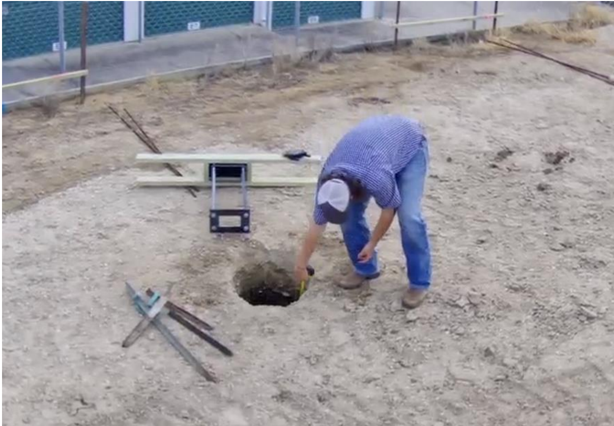
Figure 10 - Measuring of Bored Pier Depth
