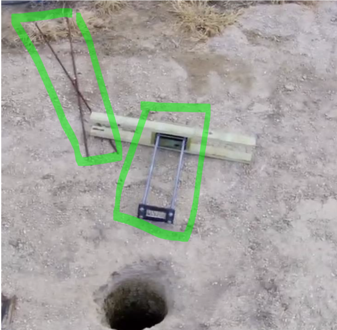
Figure 12 -Hold Down Bolts and Reinforcement Bars
