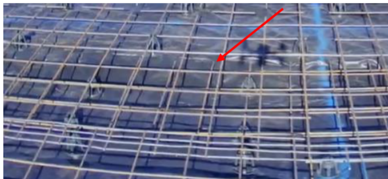
Figure 16 - Additional Bottom Mesh to Thickening
