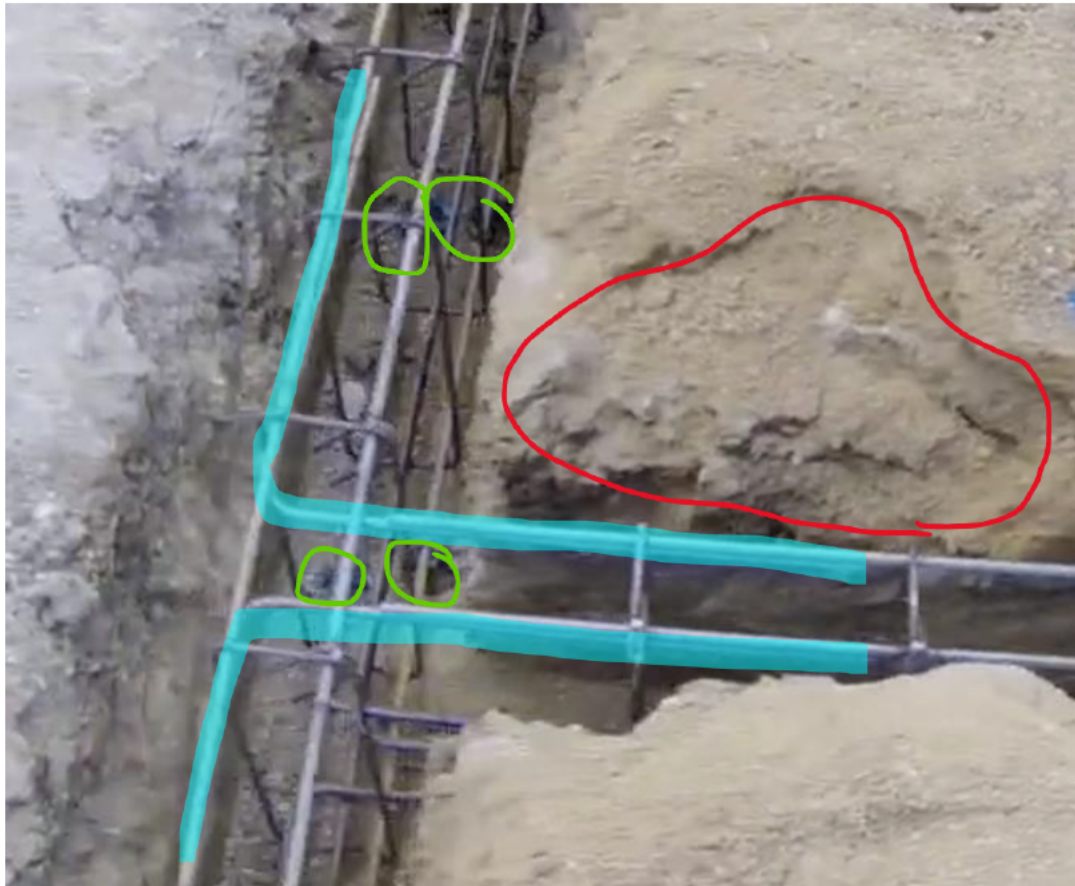
Figure 20 - Notated Image of Foundation 'T' Intersection
