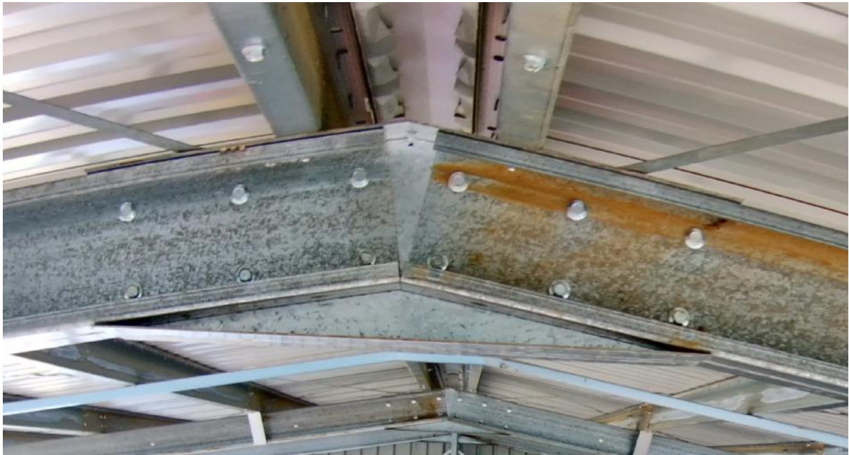
Figure 34 - Apex Connection
