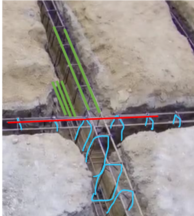
Figure 19 - Notated Image of Foundation Intersection
