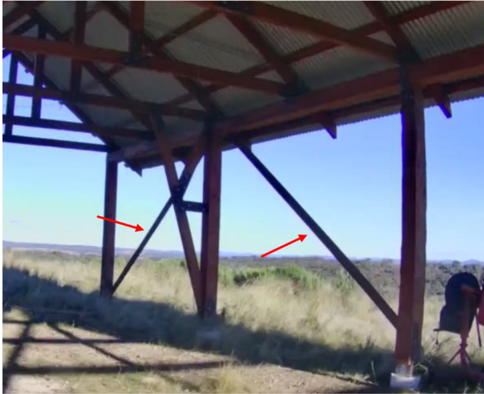
Figure 28 - Brace Sets and Columns
