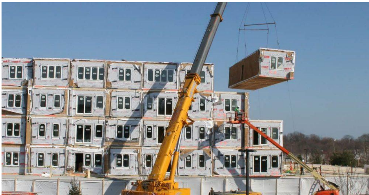
Figure 2.1: Modular Construction of an Apartment Block (Ausco 2018)
