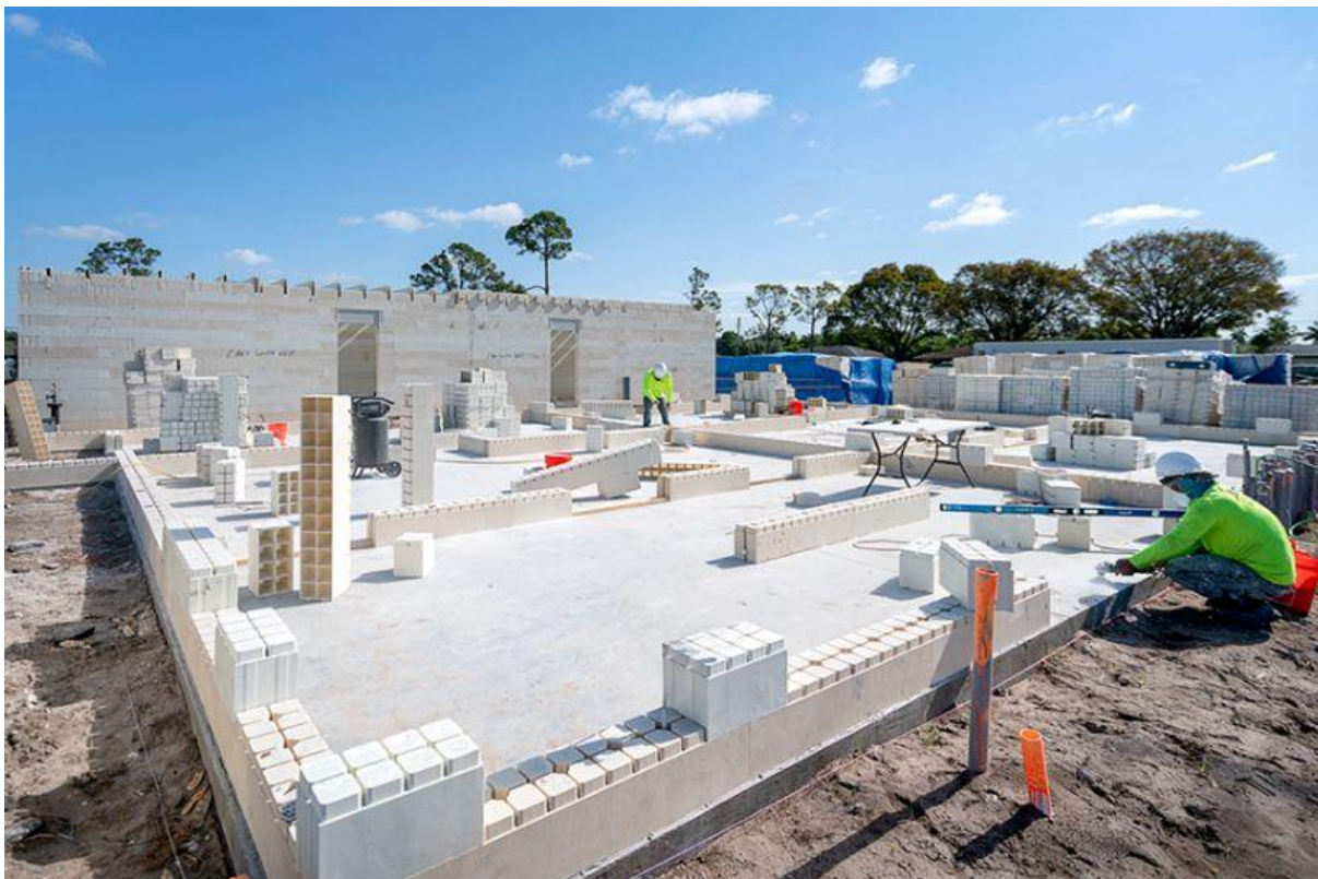
Figure 2.8: Renco Interlocking Blocks (Built Offsite, 2014)
