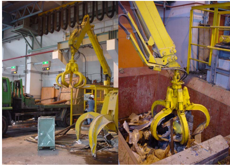
Figure 1.3.1.3: Overview of Screening Bulky Waste at the Refuse Reception Hall
