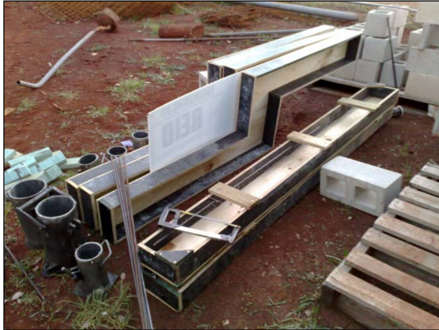
Figure 3.10 Constructed formwork.
