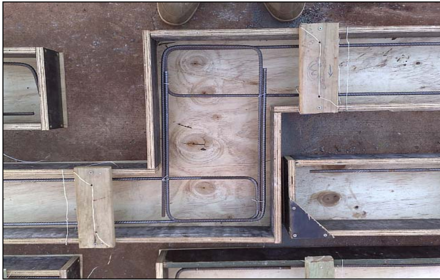
Figure 3.12 Reinforcing support and positioning.
