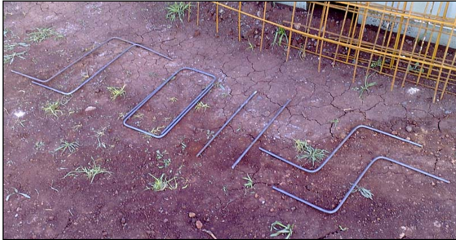
Figure 3.11 Step envelope reinforcing.
