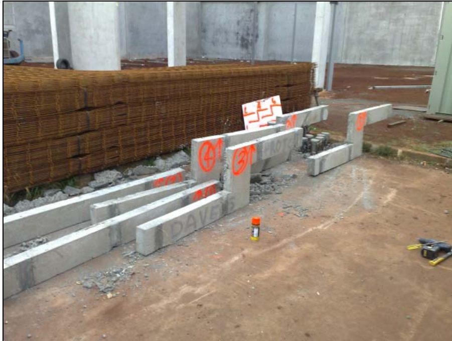
Figure 3.13 Finalised beam construction.
