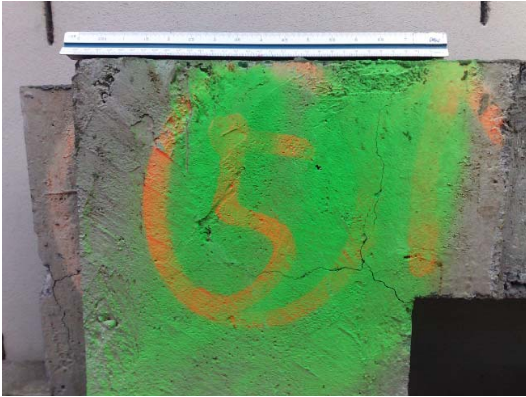
Figure 4.12 Beam 5 crack patterns.
