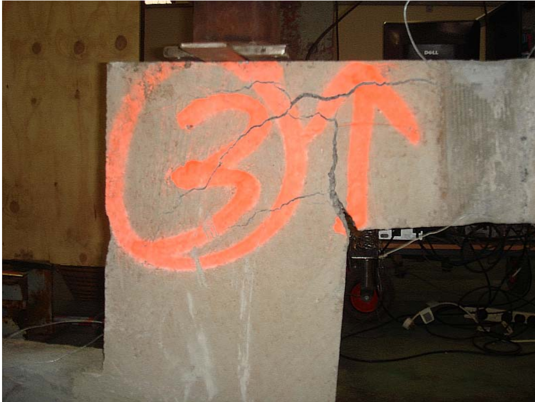
Figure 4.6 Beam 2 crack patterns.
