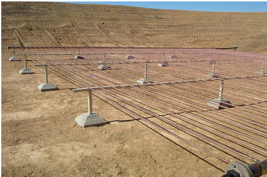
**Figure 2.6** Installed Cooling Grid, *Source: DNR&W*
