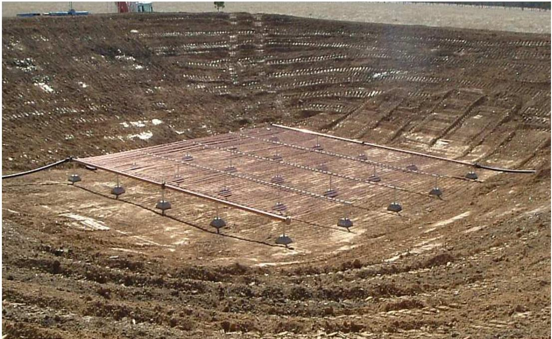
**Figure 2.5** Installed Cooling Grid, *Source: DNR&W*
