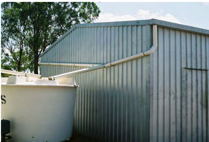
Figure 3.3 Aurukun Power Station – Line store and tank
