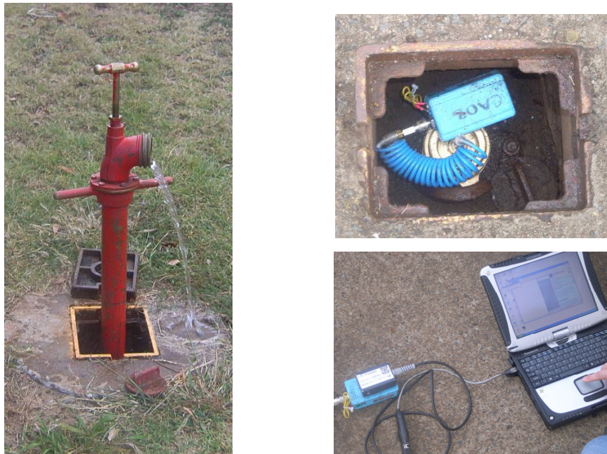
Figure 3-5 Pressure logging. Flushing (left), hydrant cap and logger in place (top right) and reading the logger (bottom right)
