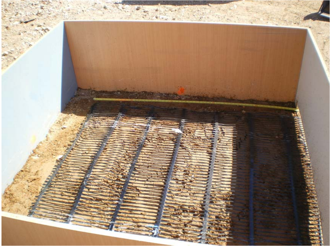
Figure 10 Placing the Tensar Geogrid 40RE
