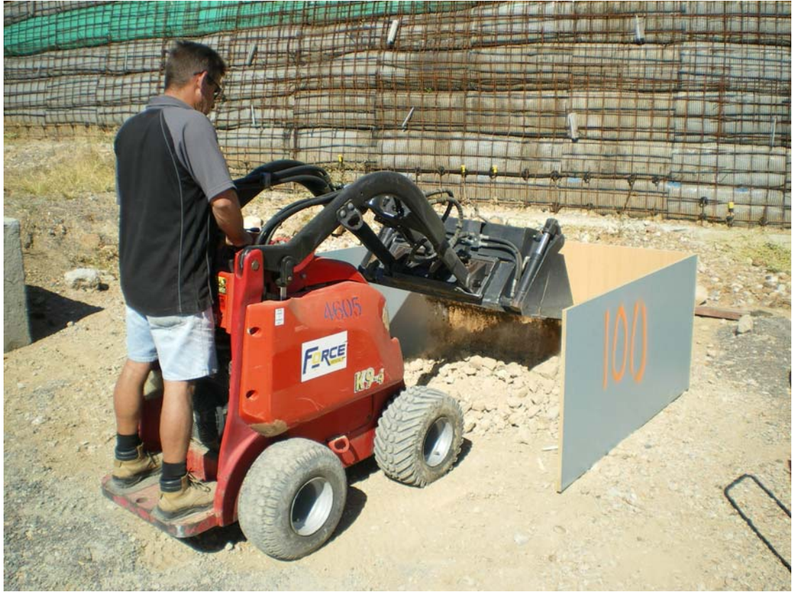
Figure 8 Placing the 100mm minus Material
