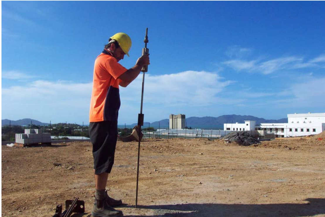
Figure 12 Dynamic Cone Penetrometer Testing
