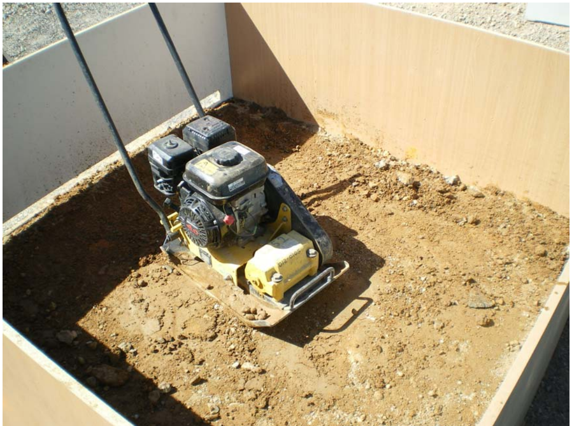
Figure 9 Compaction of the Crushed Concrete Material with a Vibrating Plate
