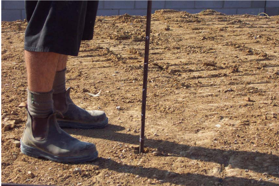
Figure 13 Dynamic Cone Penetrometer Testing (Penetration of steel rod)
