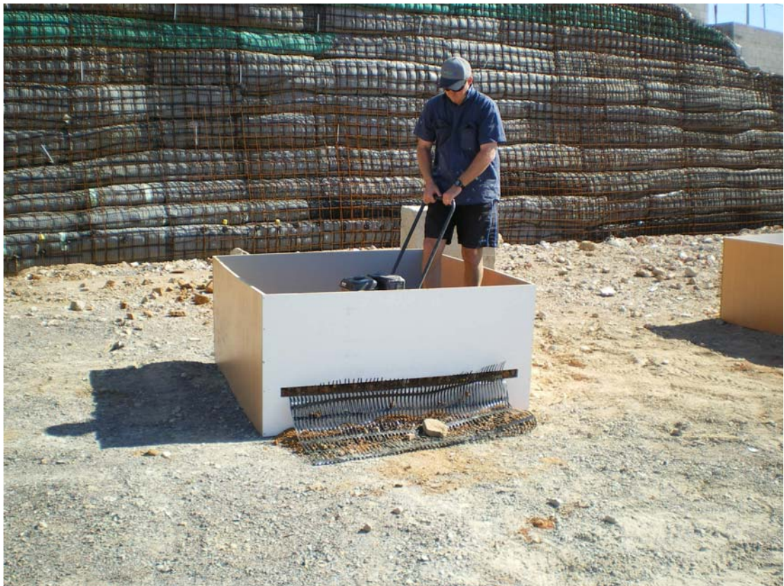
Figure 11 Finalising Material Compaction with Tensar Geogrid in Place
