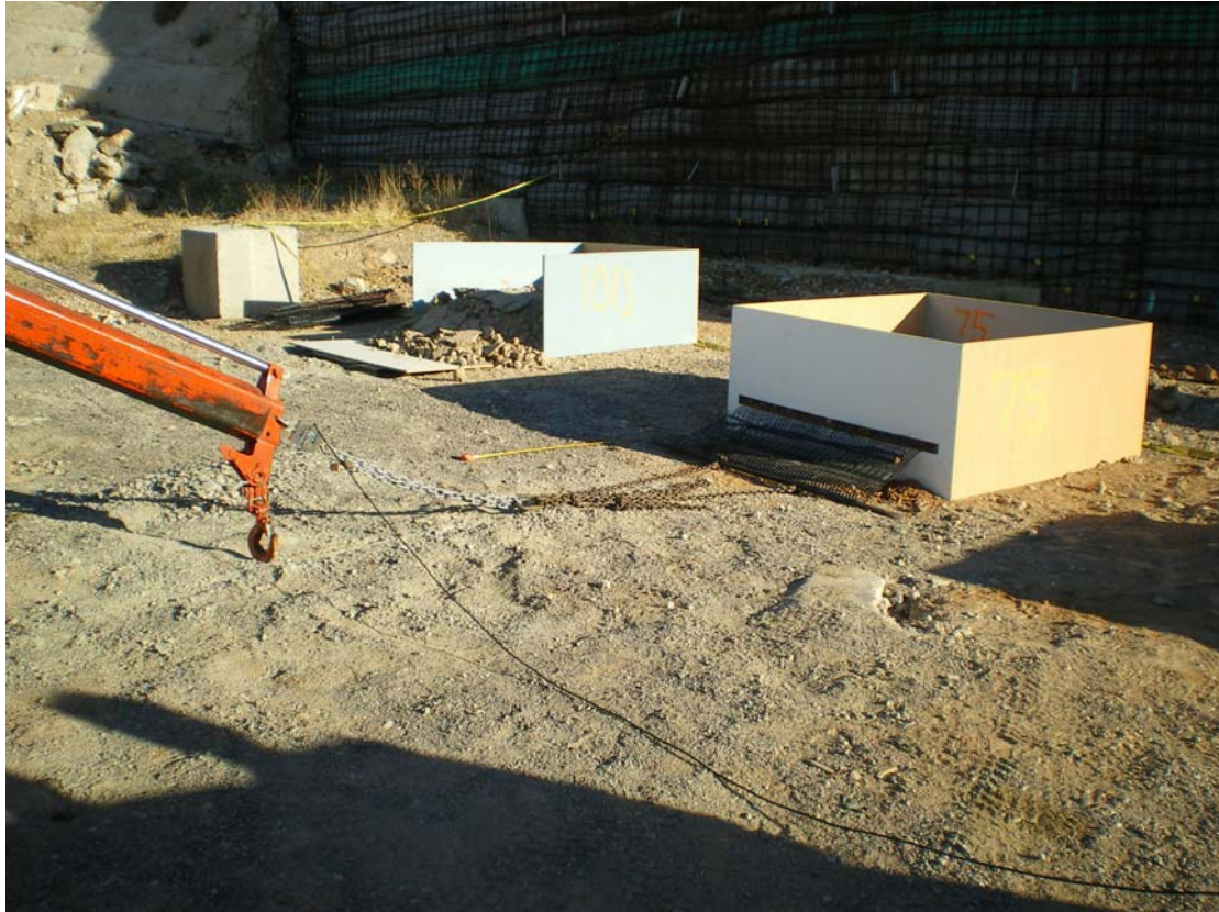
Figure 15 Tensar Geogrid attached to hydraulic arm with chains and shackles
