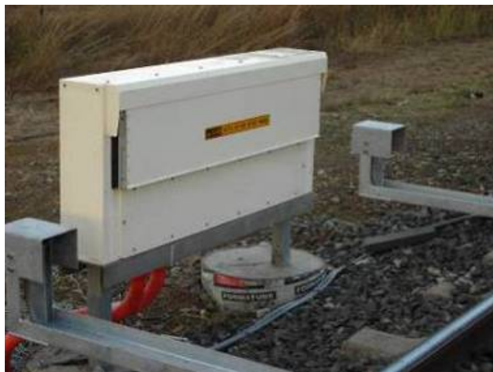
Figure 4.5 Microphone station. (Vipac Engineers)
