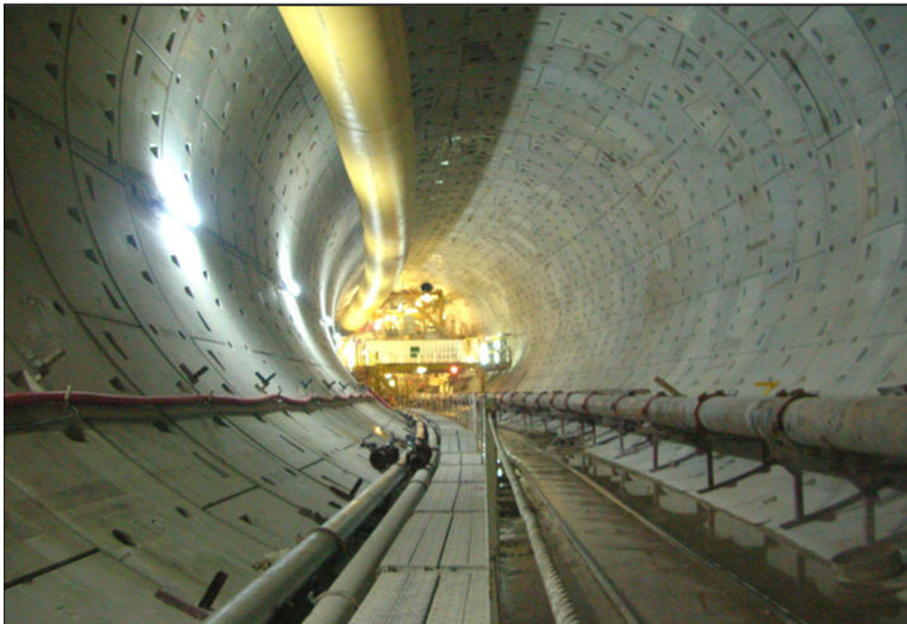
Figure 1c: SMART Tunnel boring works in progress
