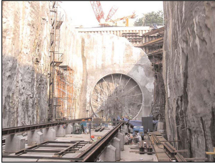
Figure 1e: TBM used in SMART Project at South Junction Box
