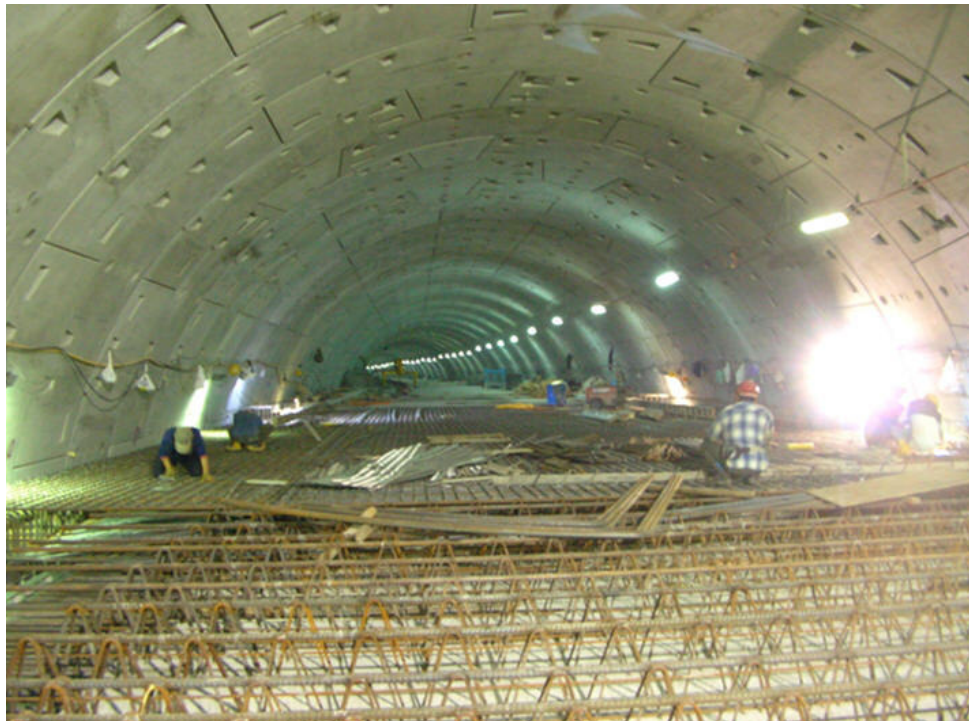
Figure 1f: Reinforcement work at upper deck
