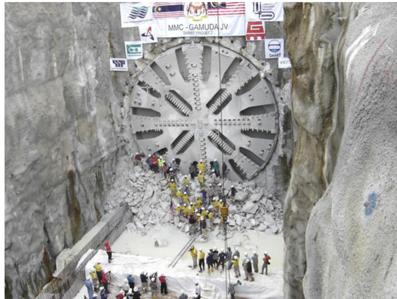
Figure 3h: TBM break through at South Junction Box
