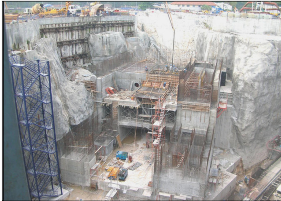
Figure 7m: Cut and fill works for SMART ventilation shaft
