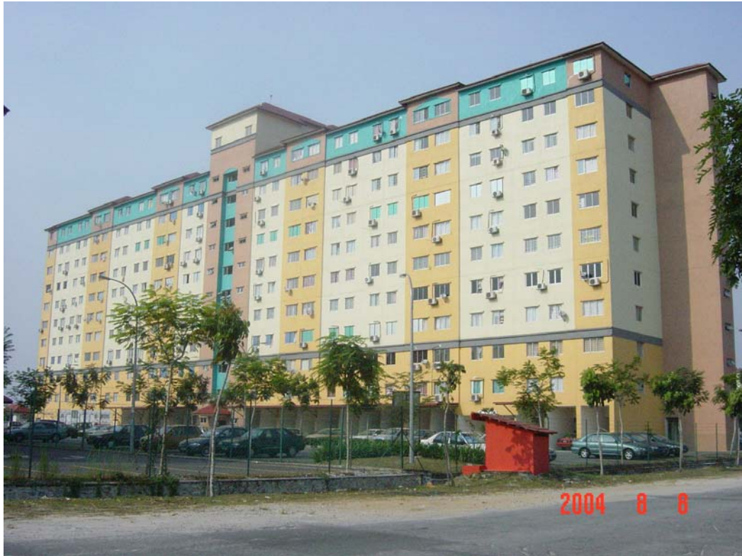
Figure 6.5: One Block of 11 Storeys Medium Low Cost Apartment.
