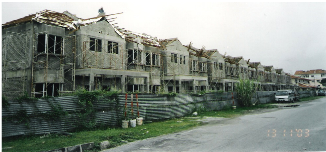
Figure 6.2: Roof Construction of Project 1 in Progress.
