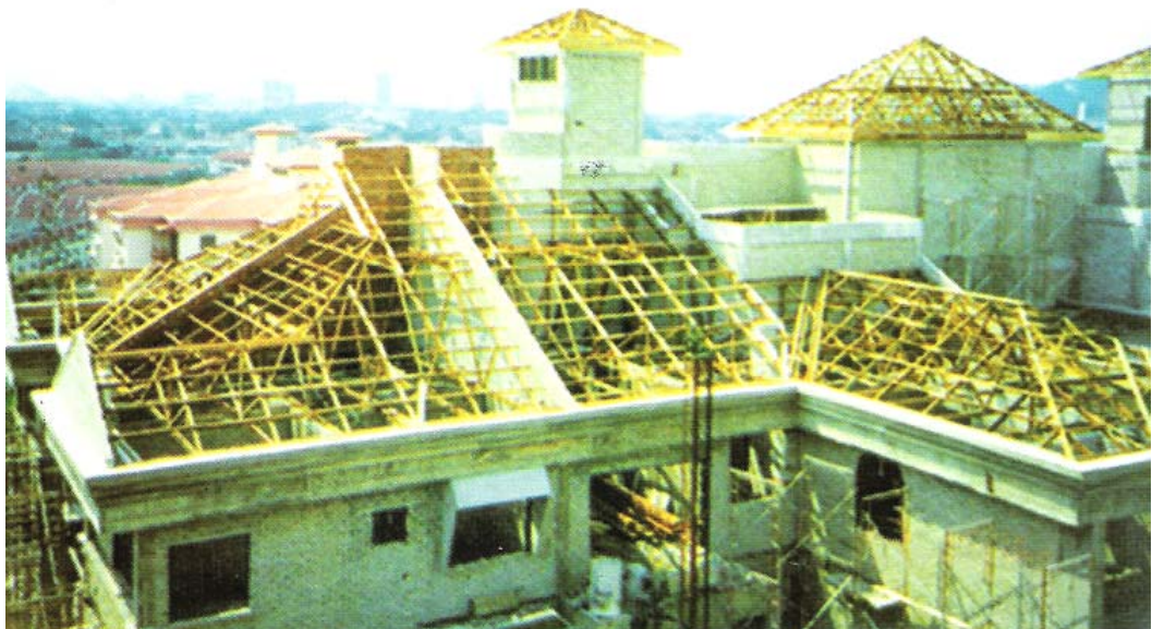
(b) Application of Timber Trusses in Condominium.
