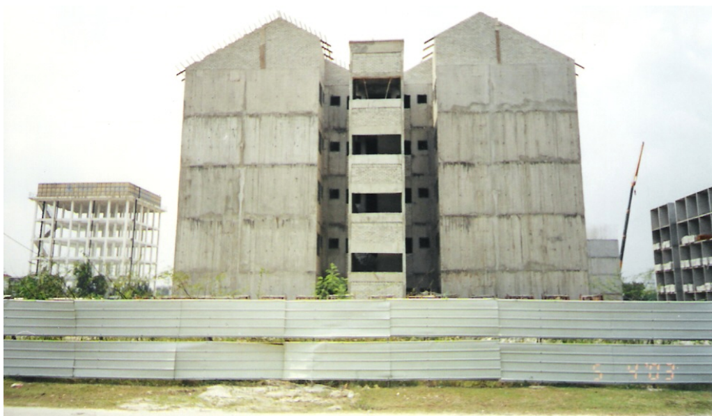
Figure 6.4: Roof Construction of Project 2 in Progress.
