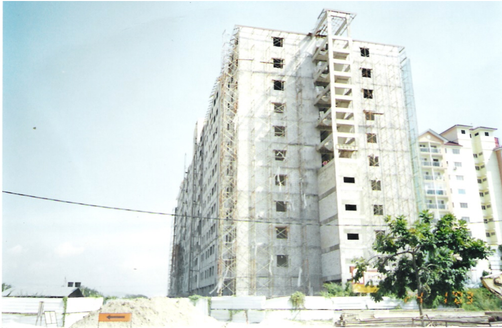
Figure 6.6: Roof Construction of Project 3 in Progress.
