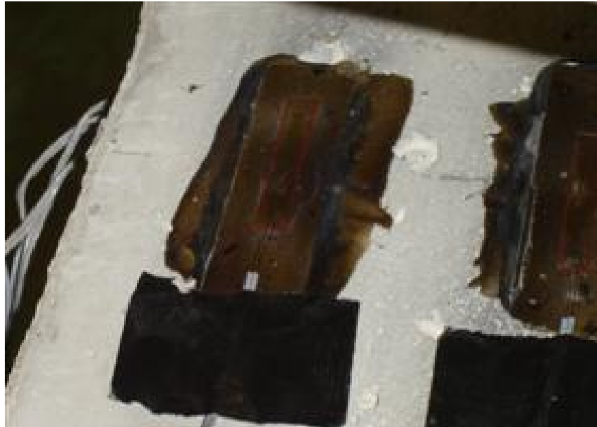
Figure 4.14: Top Concrete Strain Gauges
