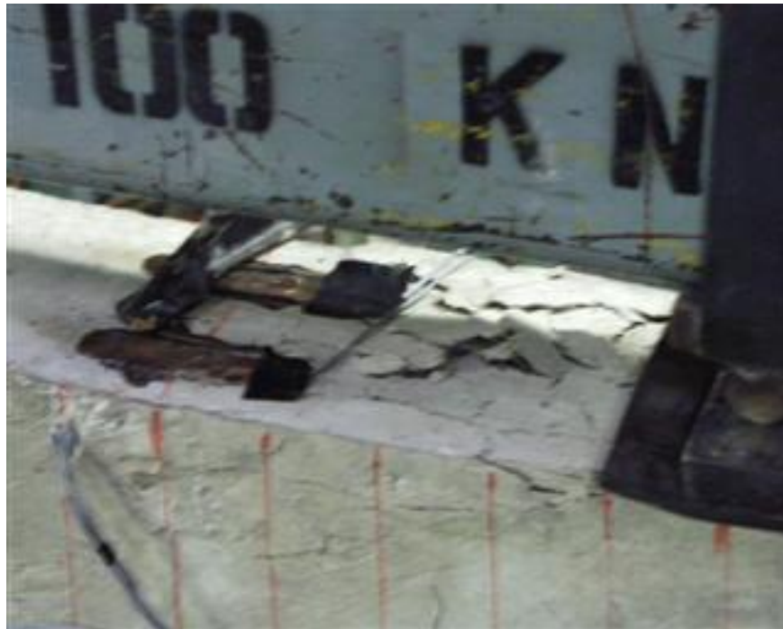
Figure 5.4: Local Crushing of the Concrete Mid-Span of the Beam
