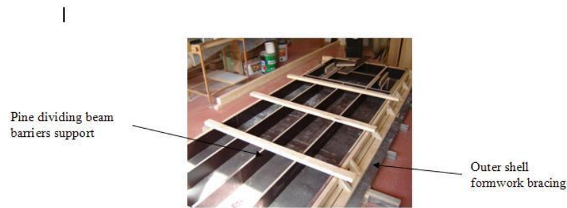
Figure 4.2: Completed Formwork
