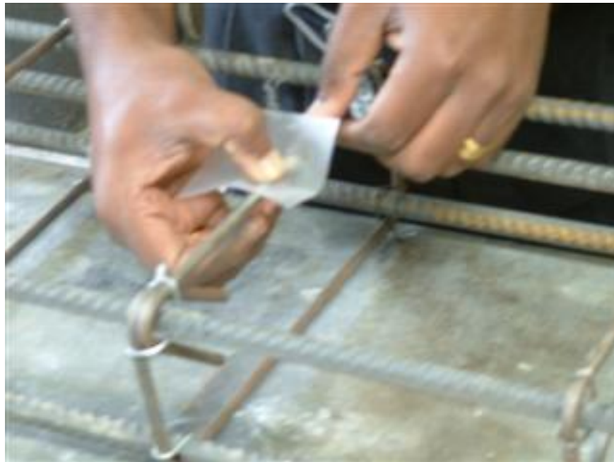
Figure 4.12: Application of Shear Reinforcement Strain Gauges
