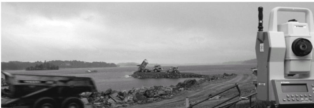
Figure 1.1: RTS being used for the guidance of scrapers. (Trimble, 2005)
