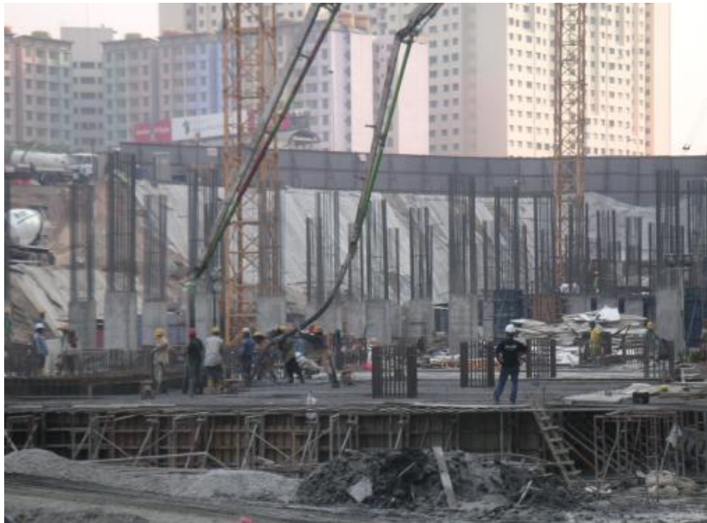
Figure 3.5: Construction of Raft Foundation-1
