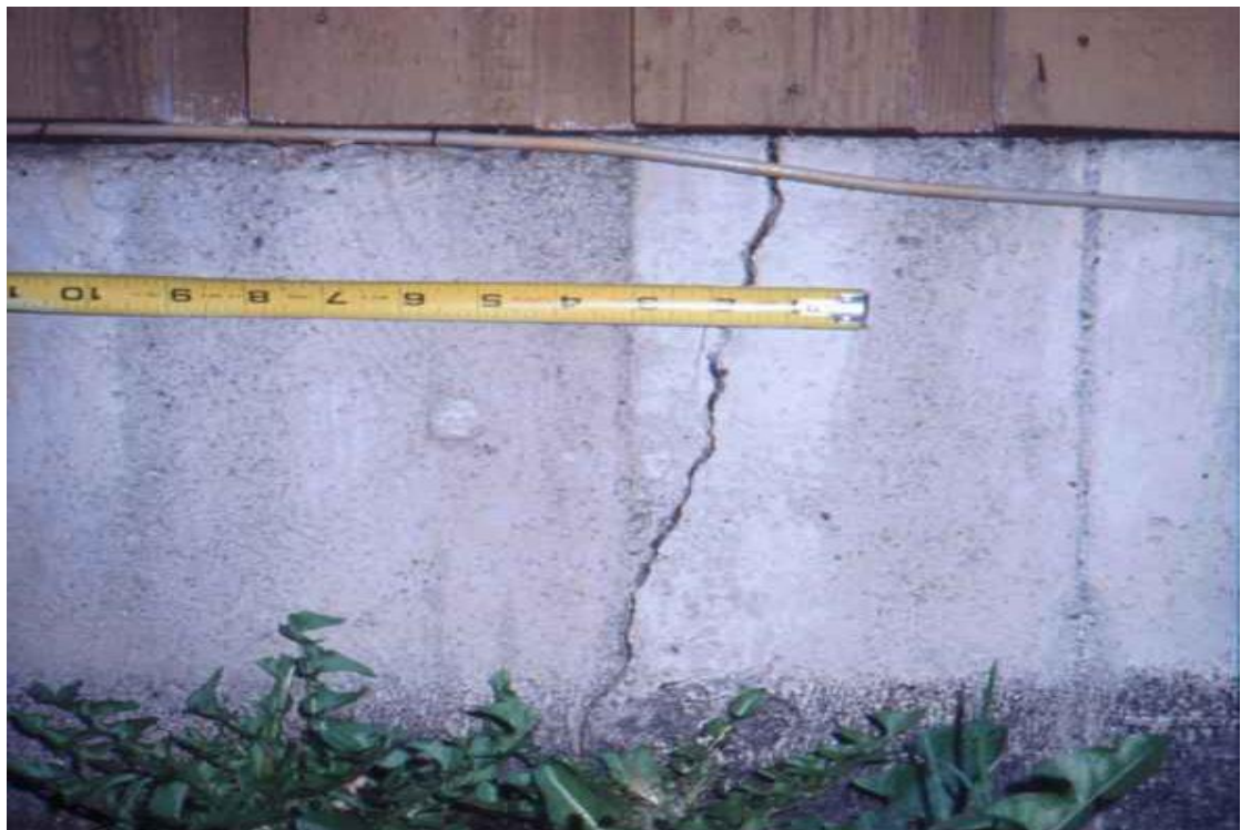
Figure 4.5: Settlement Crack
