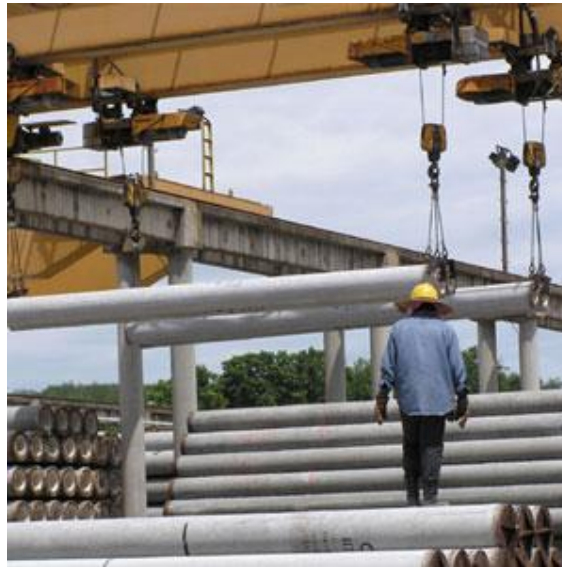
Figure 3.9: Lifting of Concrete Piles
