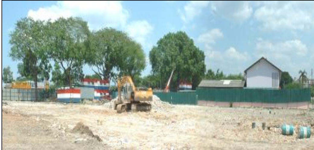
Figure 5.11: Existing Site Overview
