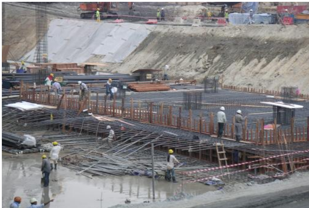
Figure 3.6: Construction of Raft Foundation-2
