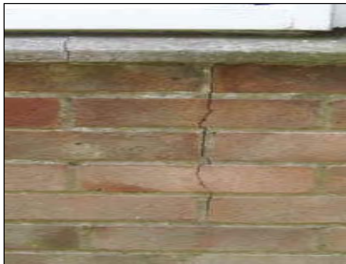
Figure 4.4: Cracks on the Wall
