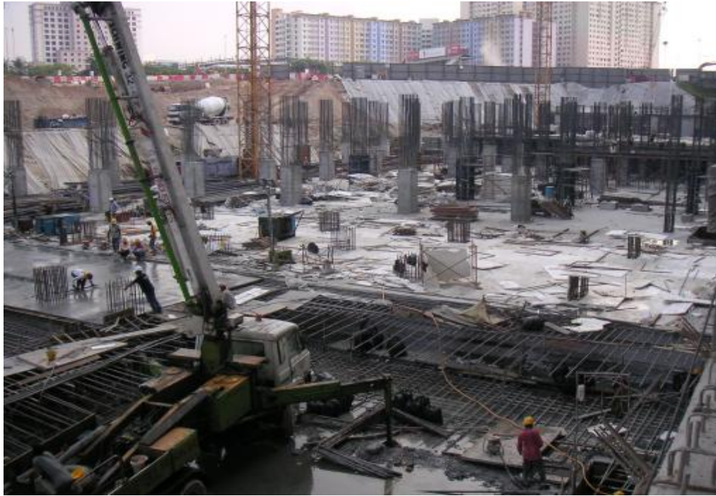
Figure 3.5: Construction of Raft Foundation-3
