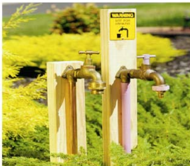
Figure 4.1 - Deliver scheme using dual reticulation pipes, recycled water delivered in lilac pipes and fittings with warning signs
