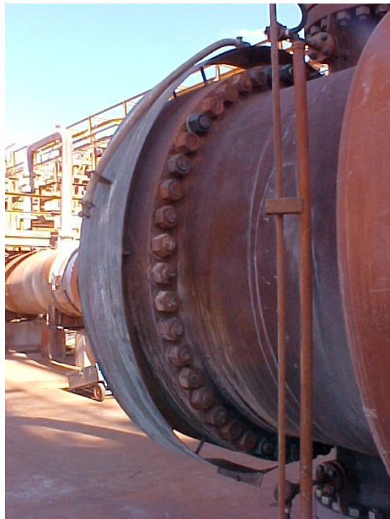
Figure 2.4 Heat Exchanger Flange Assembly [View on Flange]
