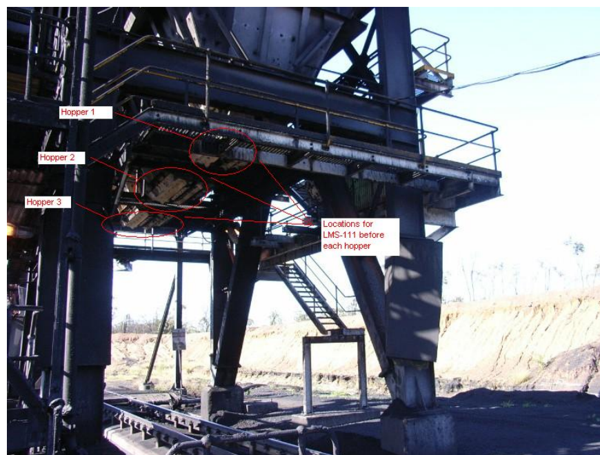
Figure 7.5: LMS-111 Locations Underneath TLO Bin
