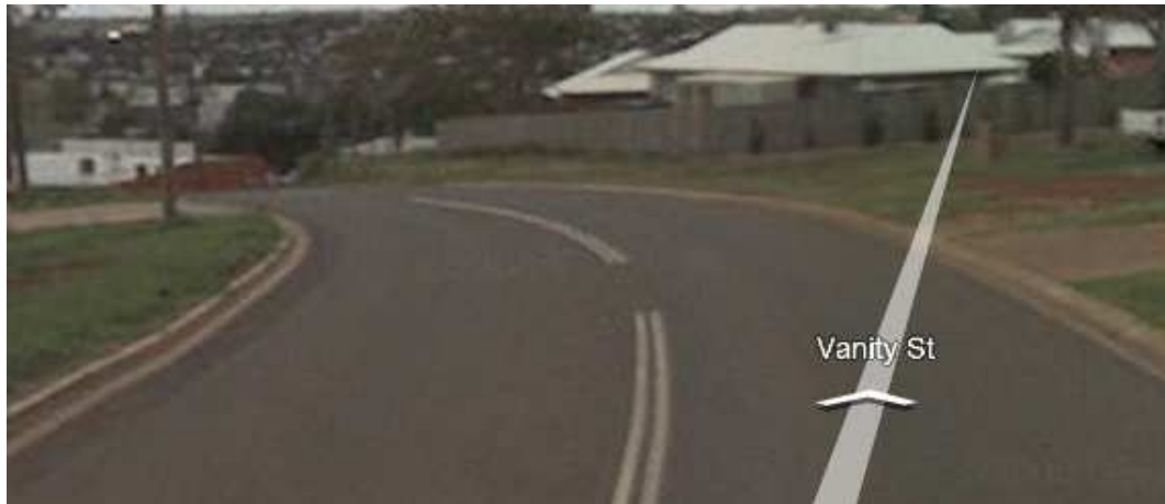
Figure 6.30 Vanity Street, Hill Approach from Top
