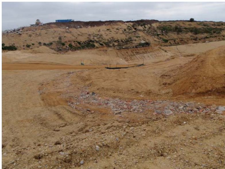
FIGURE M – PHOTO TAKEN OF SPILLWAY FROM ADDITIONAL DAM. RUBBLE SOURCED FROM ONSITE WASTE WAS USED AS BEACHING TO MINIMIZE EROSION FLOWS RUN THROUGH A DROP STRUCTURE TO THE SIDE OF ACCESS TRACK, AND THROUGH PIPE CULVERTS INTO THE LOWER (ORIGINAL) RETENTION DAM.
