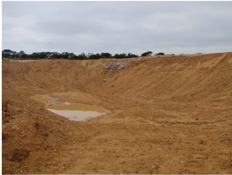
FIGURE L – PHOTO TAKEN FROM SPILLWAY OF ADDITIONAL RETENTION DAM CONSTRUCTED TO ALLOW BETTER SURFACE WATER CONTROL
