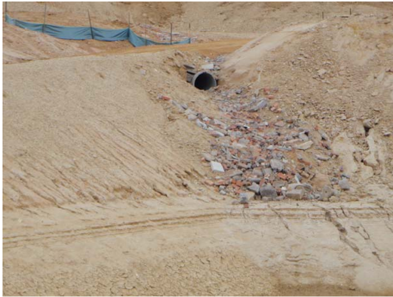
FIGURE N – PHOTO TAKEN OF PIPE CULVERT UNDERNEATH ACCESS TRACK FROM NEW RETENTION DAM SPILLWAY
