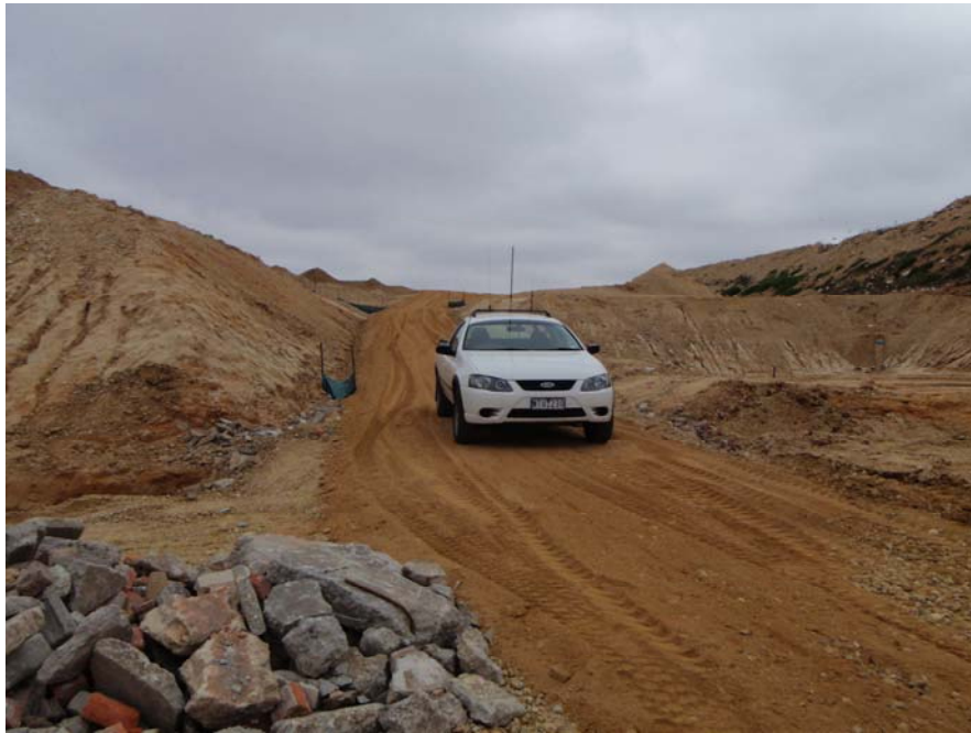
FIGURE K – PHOTO SHOWING SOME OF THE REMEDIAL ACTION TAKEN ON ACCESS TRACK LEADING INTO CELL 2. GRAVEL THAT HAS BEEN PLACED WAS STILL AWAITING FINAL COMPACTION AT THIS POINT, HAS SINCE BEEN COMPLETED. ALSO NOTE THE BUND WALL ON EDGE OF DAM.
