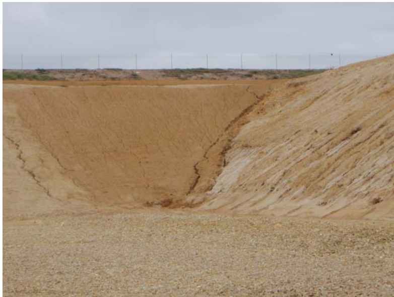
FIGURE O – PHOTO ILLUSTRATING BATTER SLOPE EROSION
