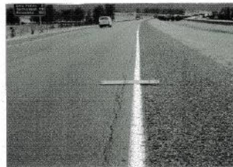
Figure 3 Longitudinal Cracking
