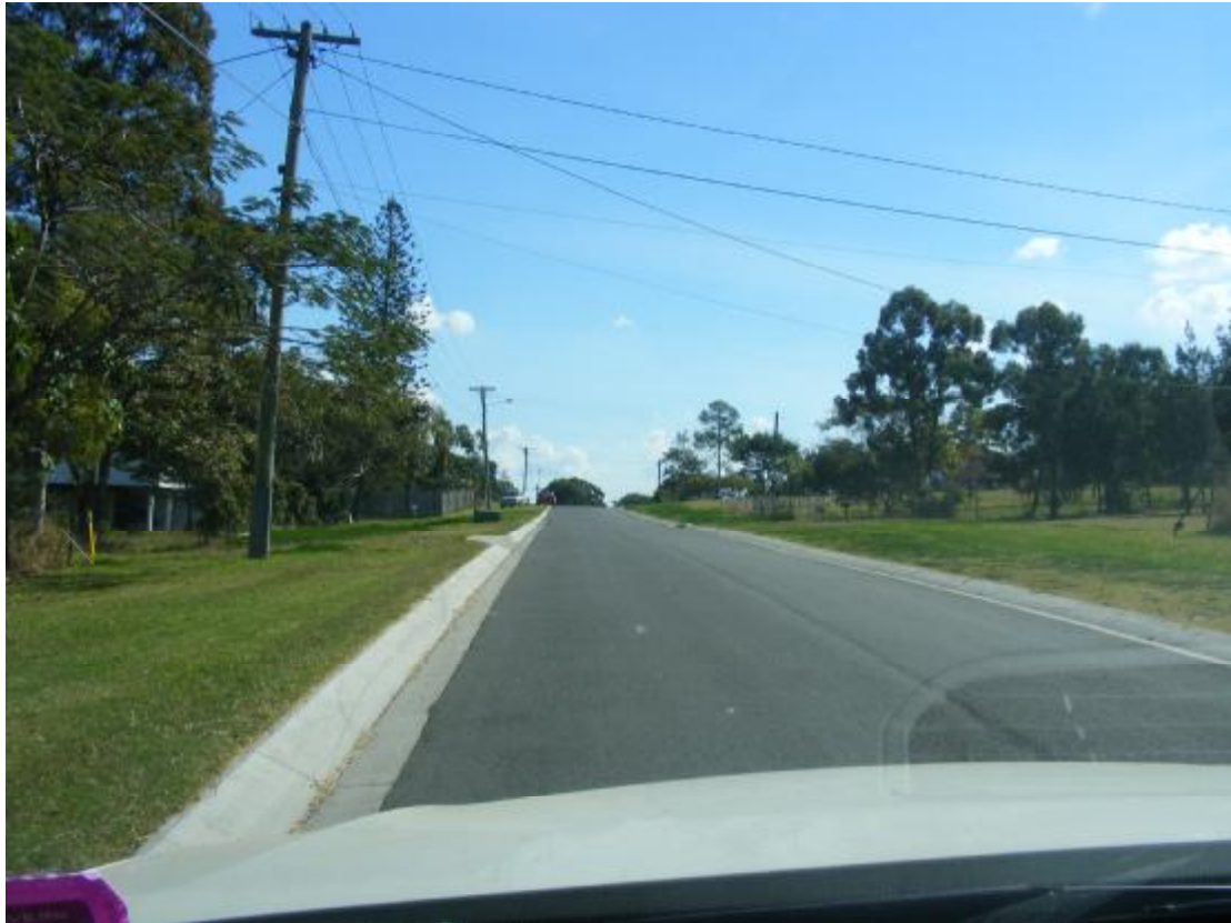
Figure 4.10: Boscawan Crescent in perfect condition
