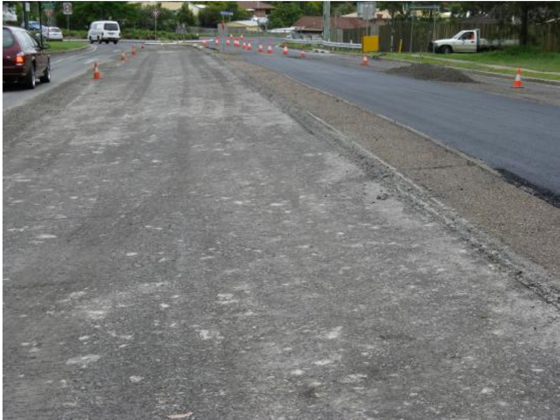
Figure 8.3: Foam bitumen treatment on Redbank Plains Road before wearing course
