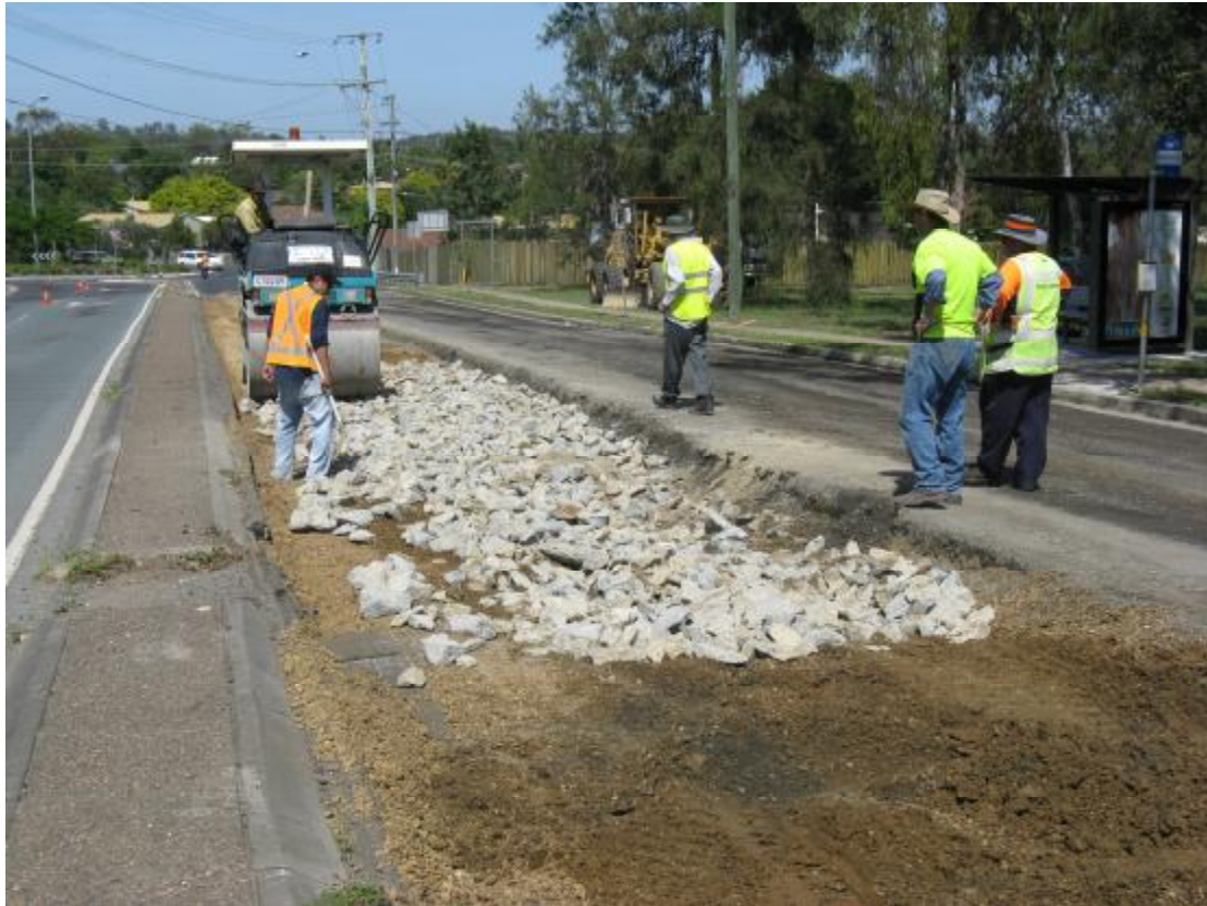
Figure 8.2. Rock stabilisation of soft subgrade
