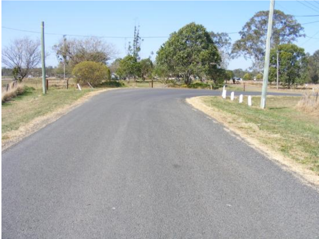
Figure 4.21: Suffield Drive section 2, good condition even on bends
