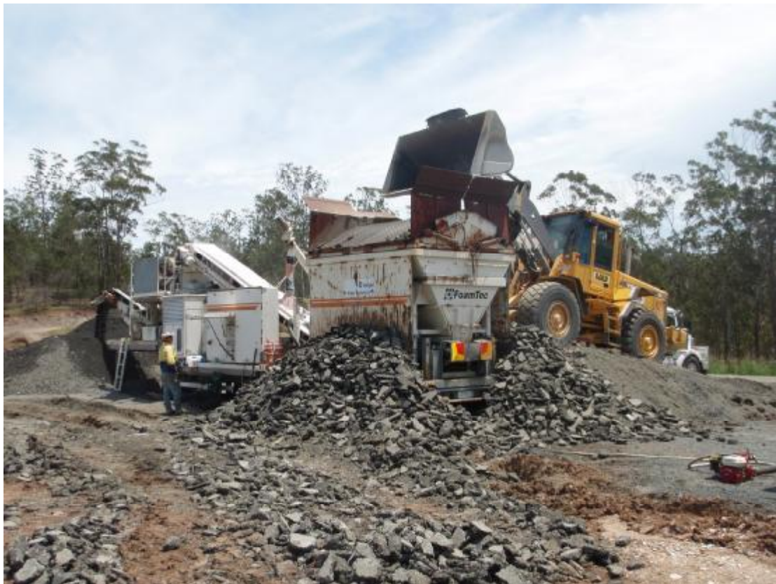
Figure 7.2: Foamed bitumen ex-situ plant producing mix
