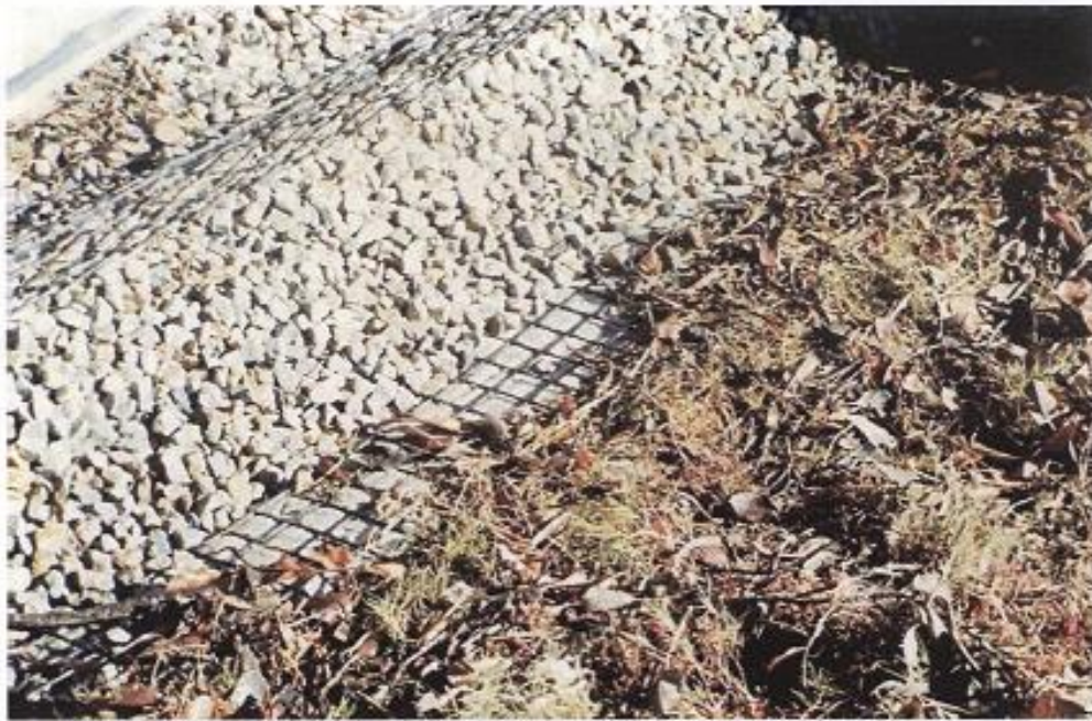
Figure 7.3: Granular platform over Tensar SS30 Geogrid (Schaeffer 2007)
