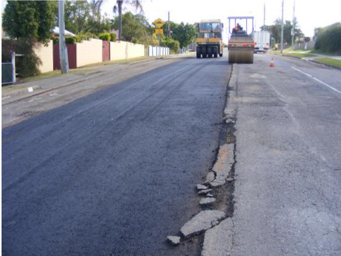
Figure 7.12: Blackstone Road Silkstone rehabilitation by deep lift asphalt
