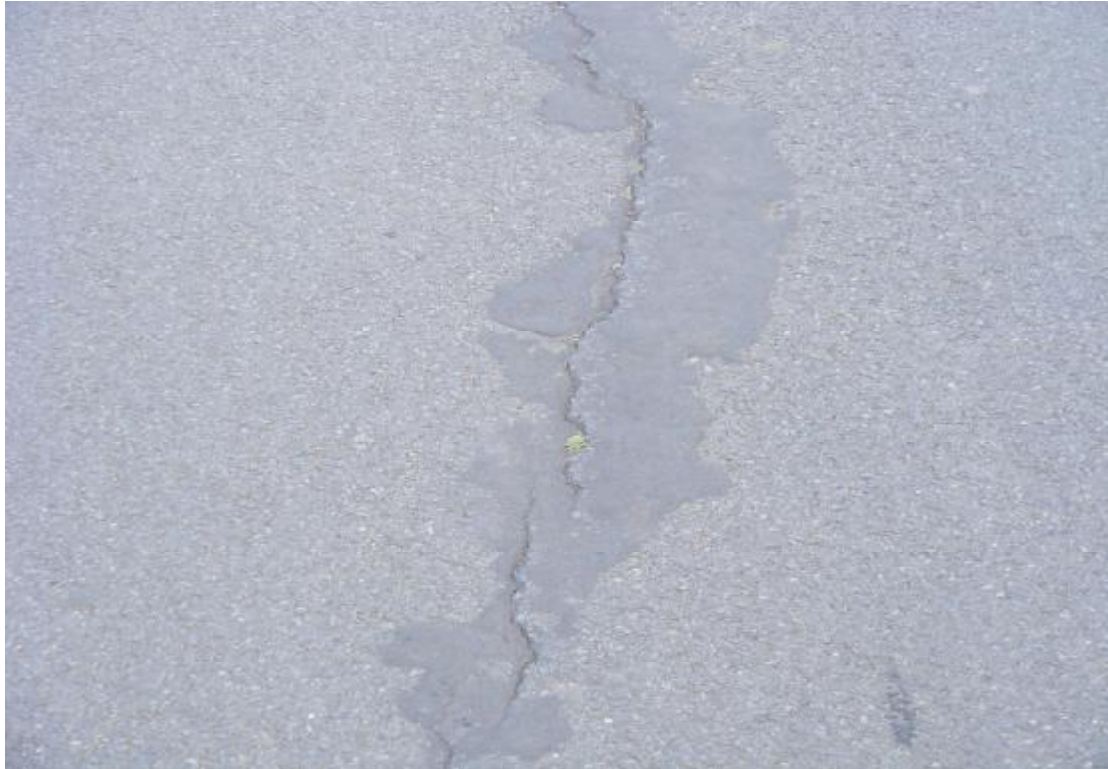
Figure 4.17: Margret Street crack sealing
