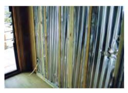
Two forms of insulation are used - radiant (aluminium foil backed felt) and bulk insulation to address extreme solar conditions of the site.
